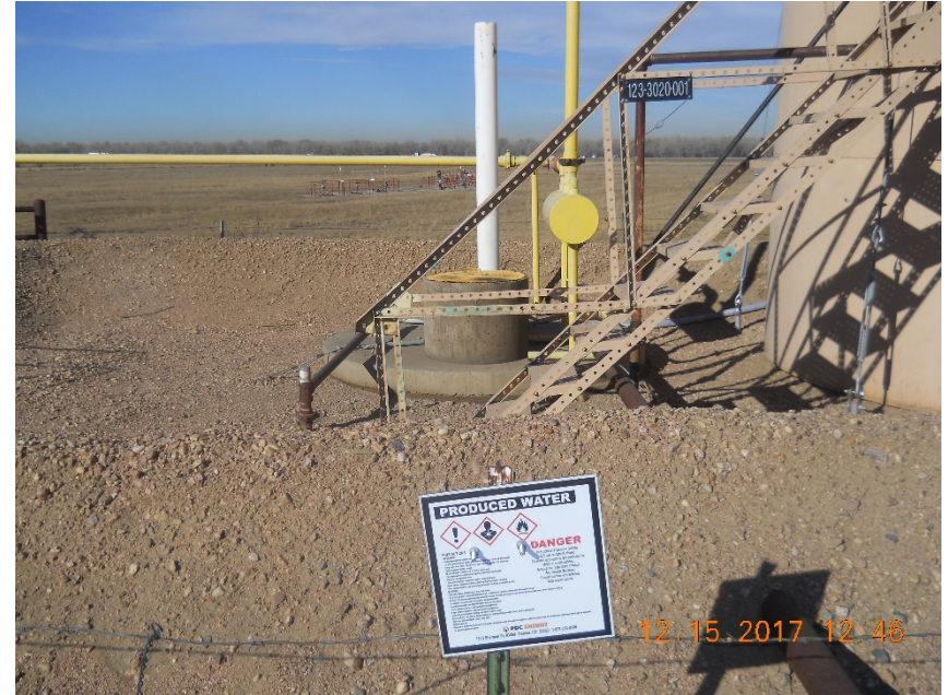
Produced water vault does not have capacity labeled and does not have NFPA placard
