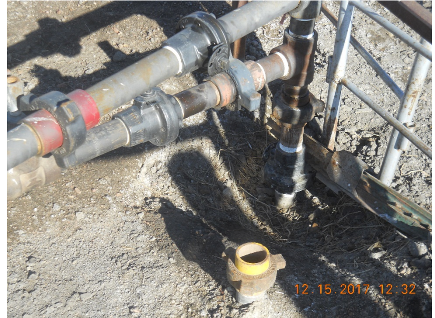
2" Balon valve from surface casing to flowline appears to be leaking. Stained soil under valve
