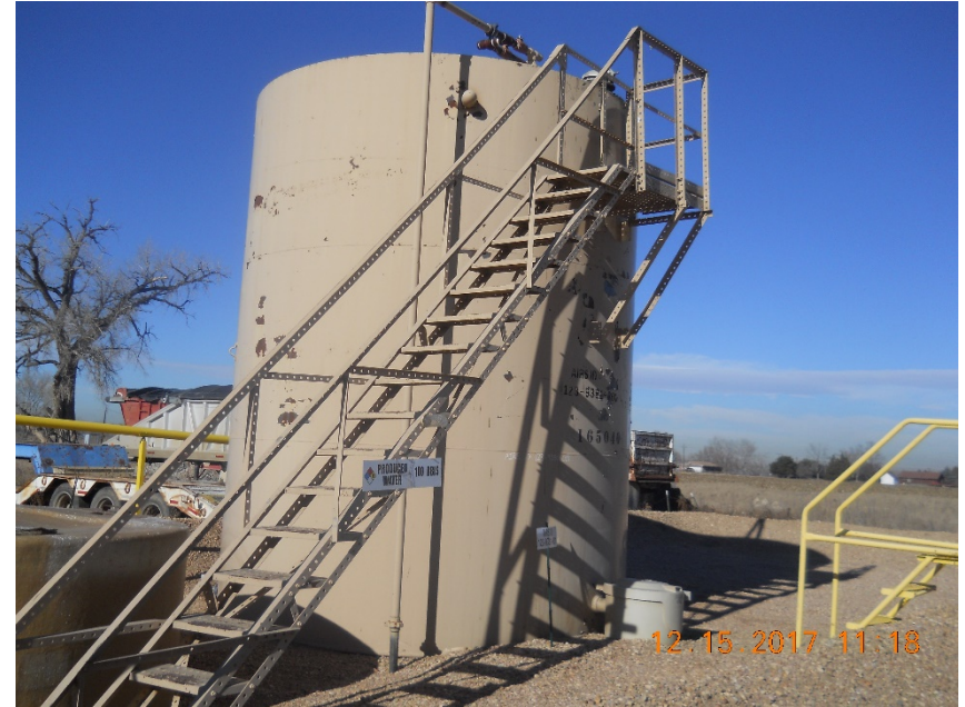
Paint is chipping on crude oil tank and has visible rust
