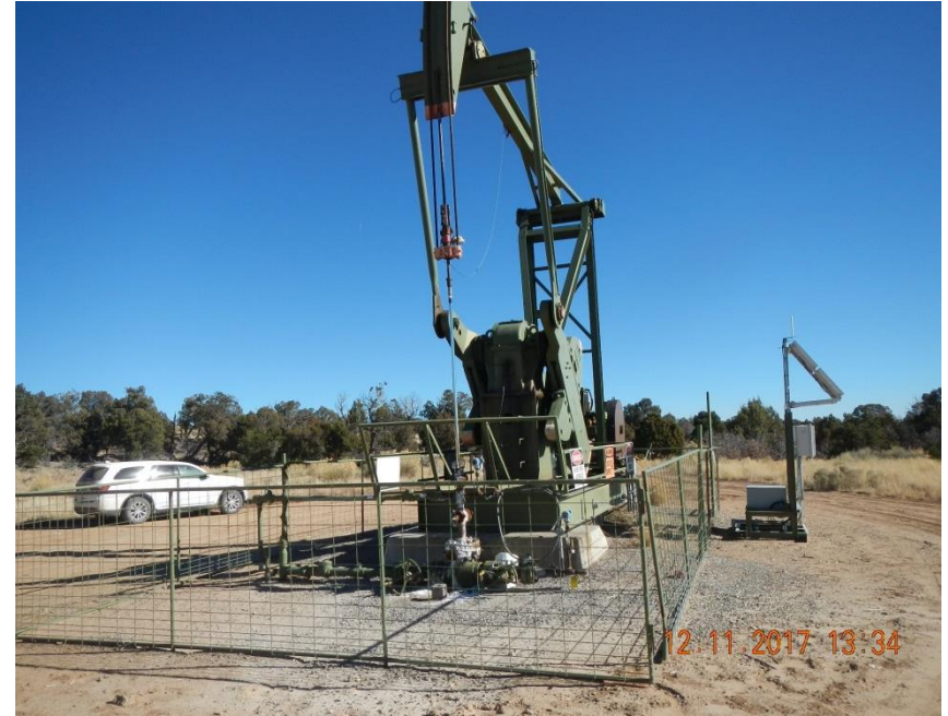
Allison Unit #147 pumping unit and well head.
