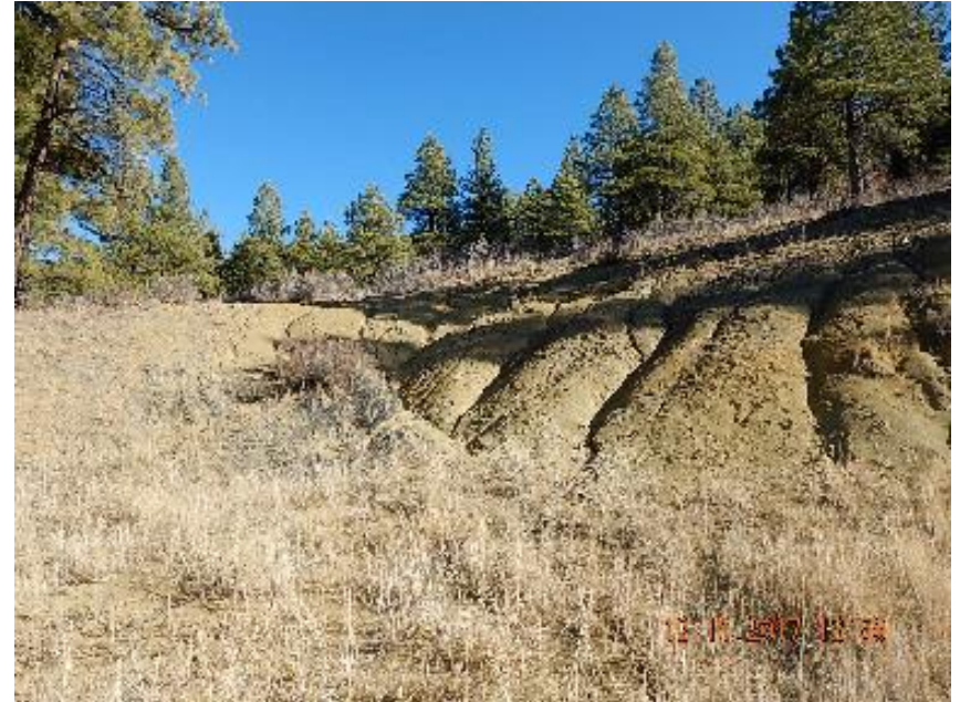
Photo 6: Erosion and rilling on the cut slope.
