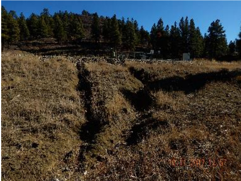
Photo 3: View of erosion channels looking from base of fill slope up towards edge of location.
