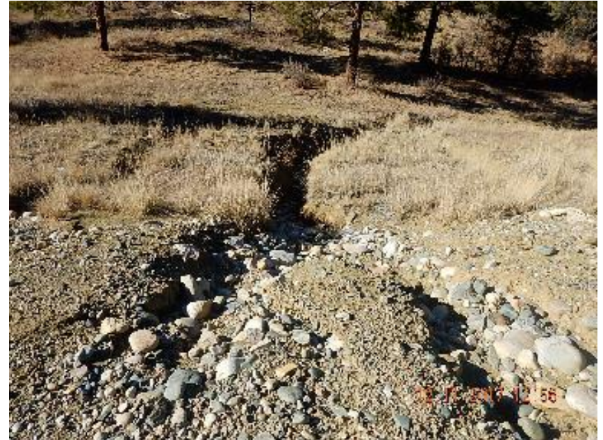
Photo 2: Erosion channel on fill slope.
