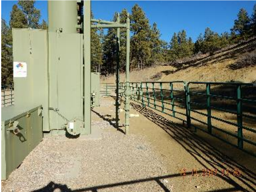
Photo 7: Sediment flowing off cut slope and into fenced production equipment area.
