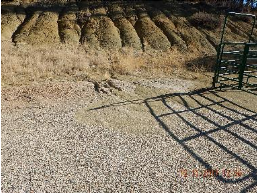
Photo 5: Breach in berm with erosion channels and rilling on the cut slope in the background.
