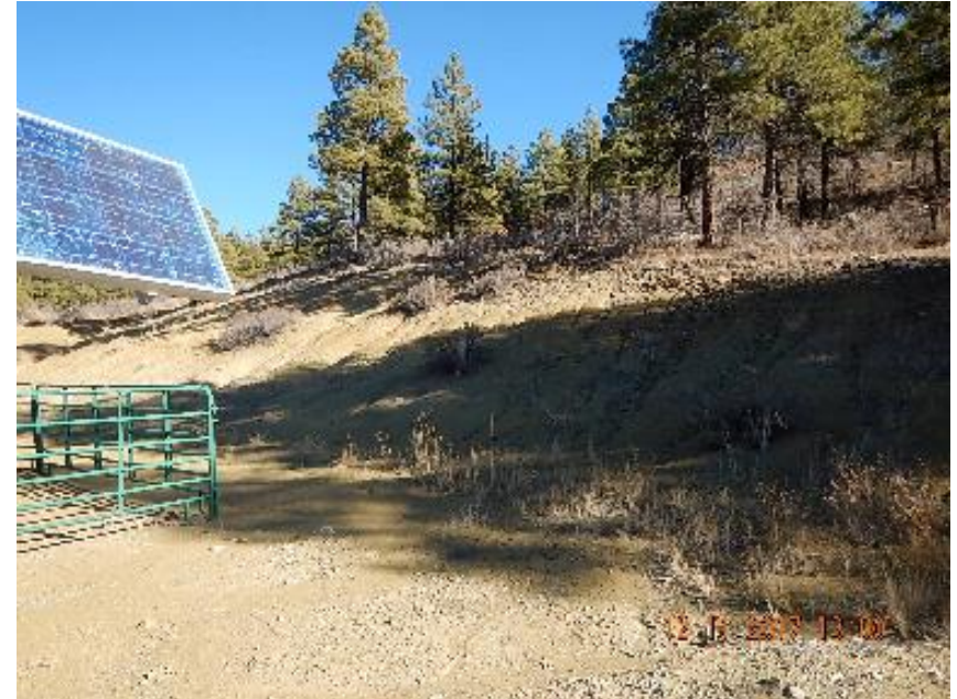
Photo 8: Erosion and rilling on the cut slope and sediment flowing down off hill towards location entrance.
