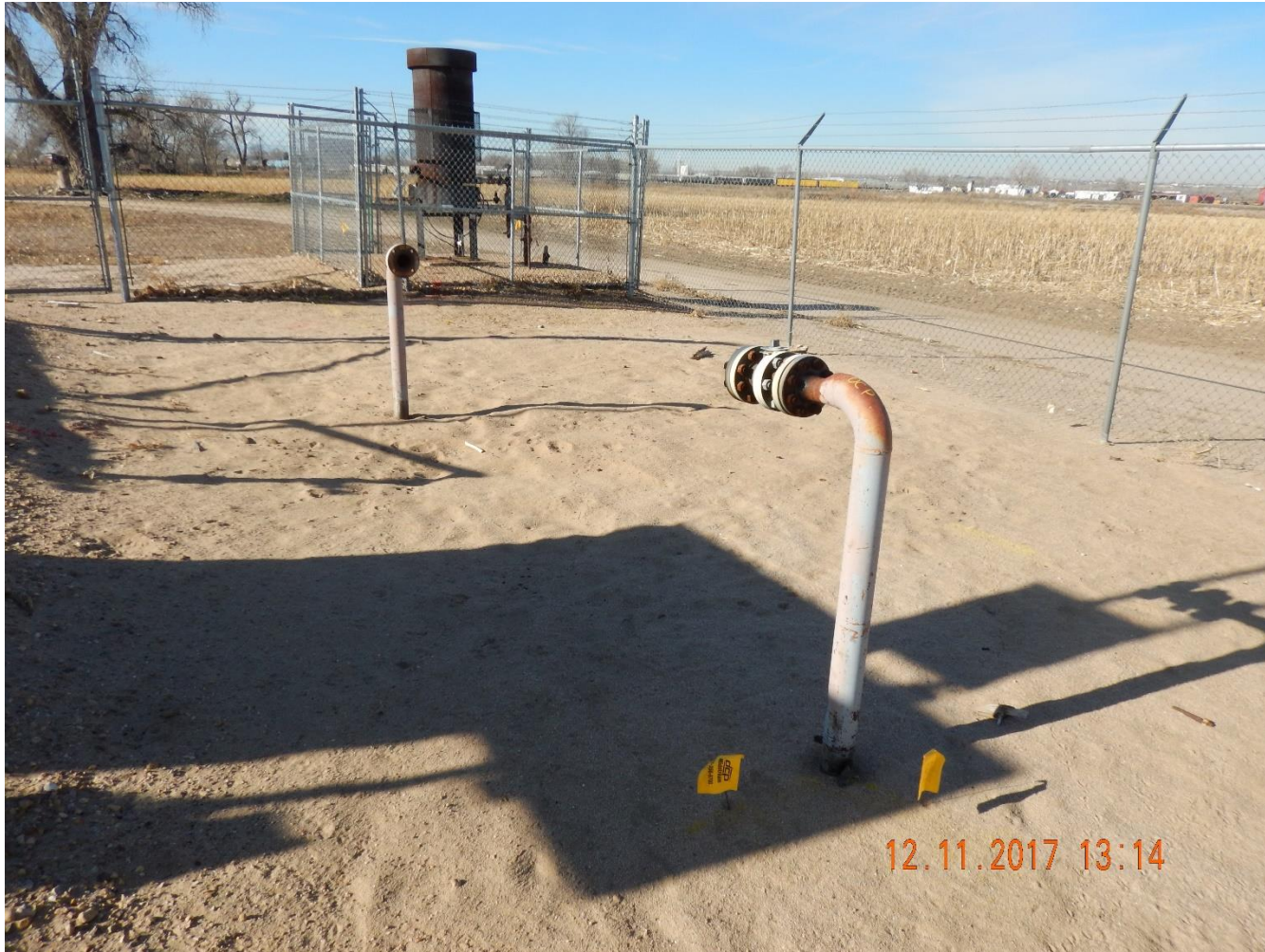
Photo 1: Photo taken from the battery location, facing west. Previous inspections required operator to remove four (4) pipe risers on the battery location in accordance to reclamation rule 1004.a. Photo shows two risers have been removed, however two risers remain on the location.
