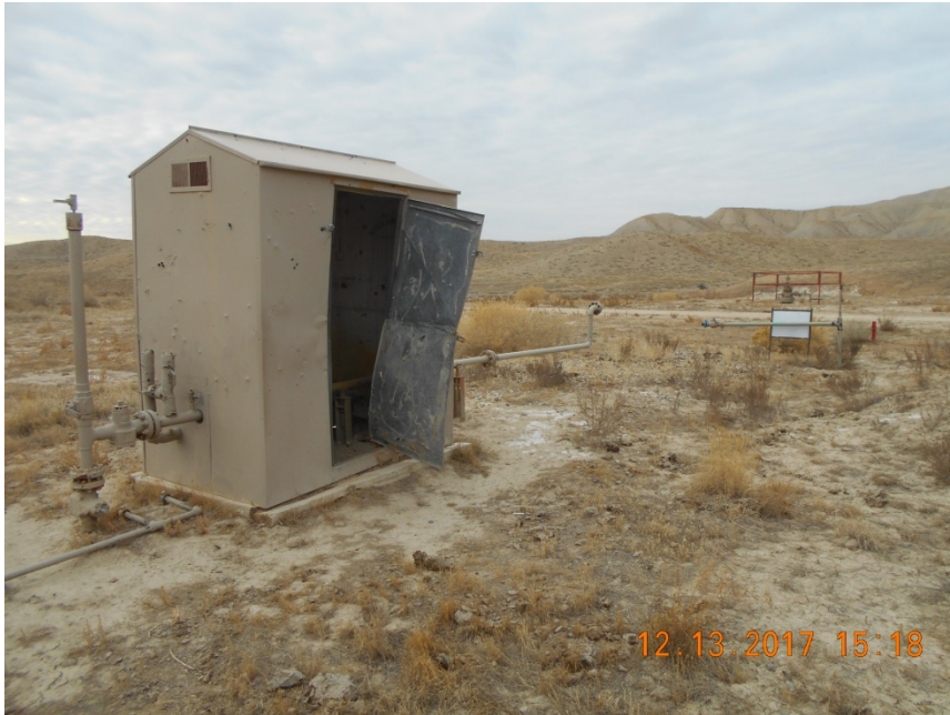
Meter housing with unused/unmarked risers and junk pipe.
