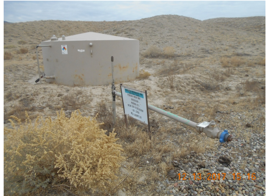
Tank battery with sign and locked out/tagged out riser.
