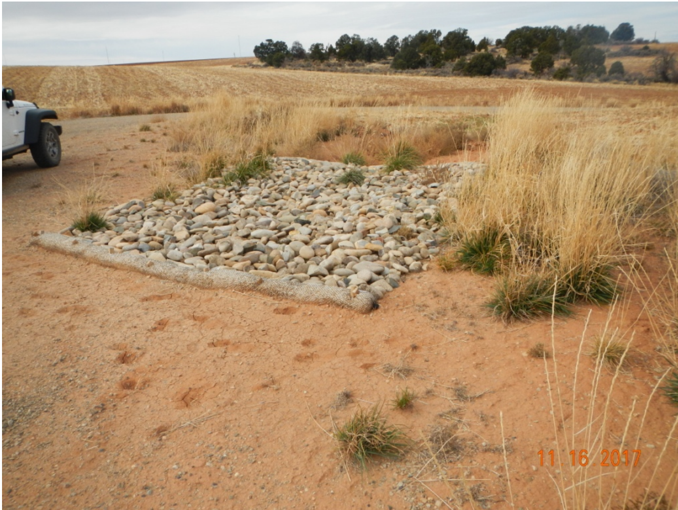
Photo 4. View of stormwater controls at the entrance to the well pad.
