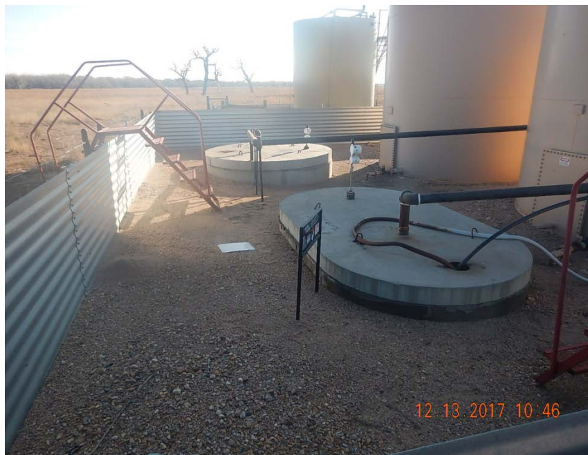
Photo 3: Vaults not anchored in floodplain.
