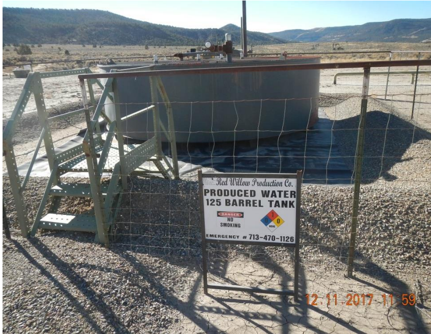
125 bbl. open topped produced water vessel that replaced 500 bbl. AST.
