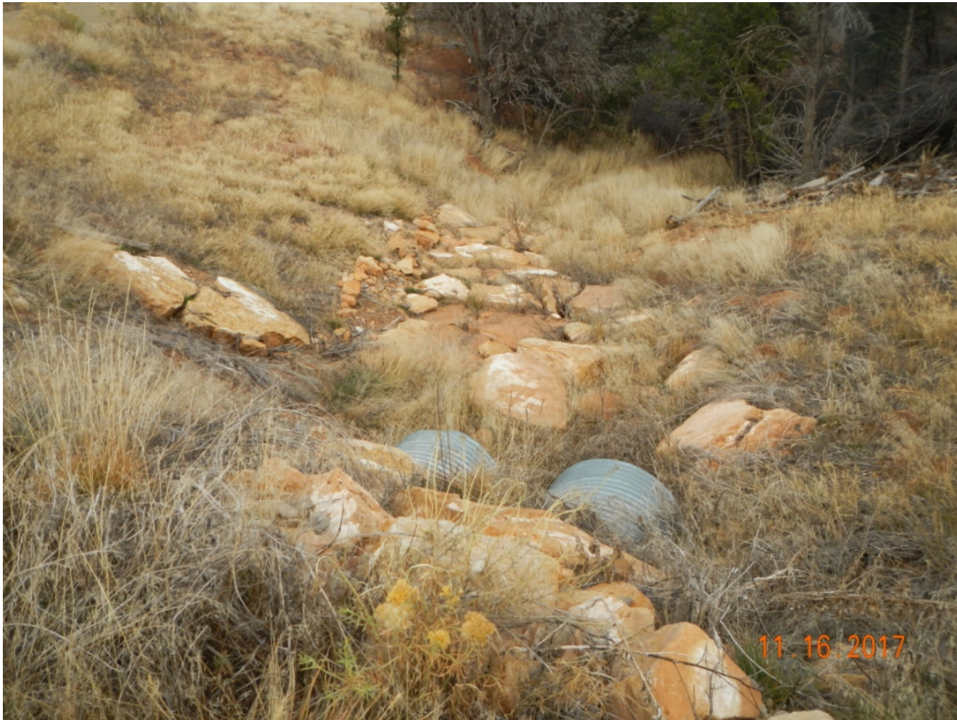
Photo 4. View of stormwater controls on the access road that appear to be functioning.
