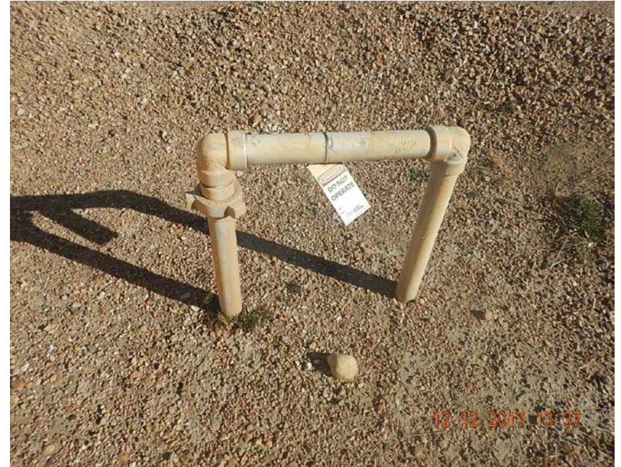
Photo 4: Deactivated riser SE of separator
