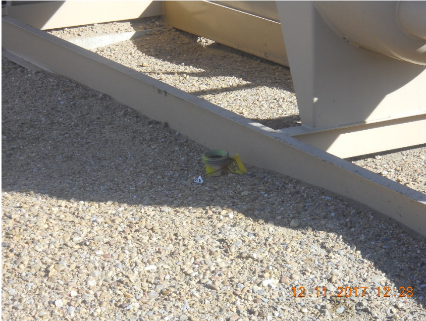
2" steel marked riser west side of separators
