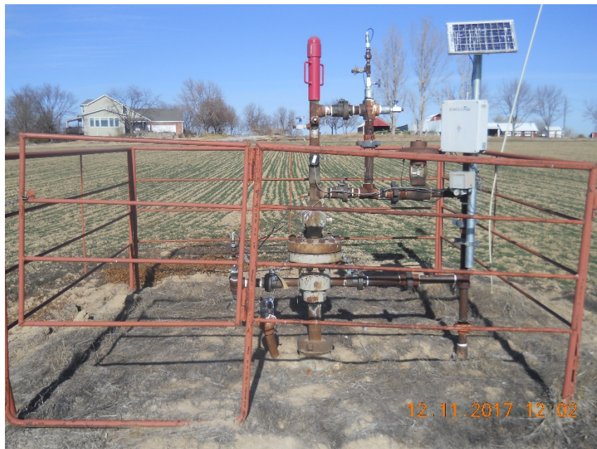
Wellhead looking north. No wellhead signage, no emergency contact information
