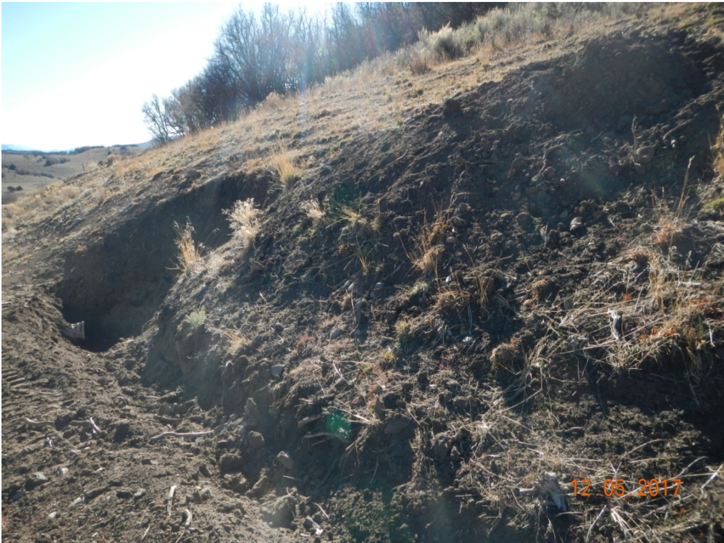
Photo 2. View of culvert inlet at that was recently cleaned, and sediment placed adjacent and up-slope from the access road. This disturbed soil will erode back to the roadside drainage and expands the disturbance, and needs to be properly managed.
