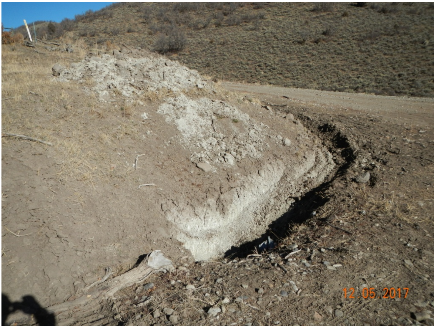
Photo 3. View of area along the access road where sediment and soil has been scraped and placed up-slope of the roadside drainage. Exposed sediment will rapidly erode, and this practice expands project disturbance by smothering vegetation.
