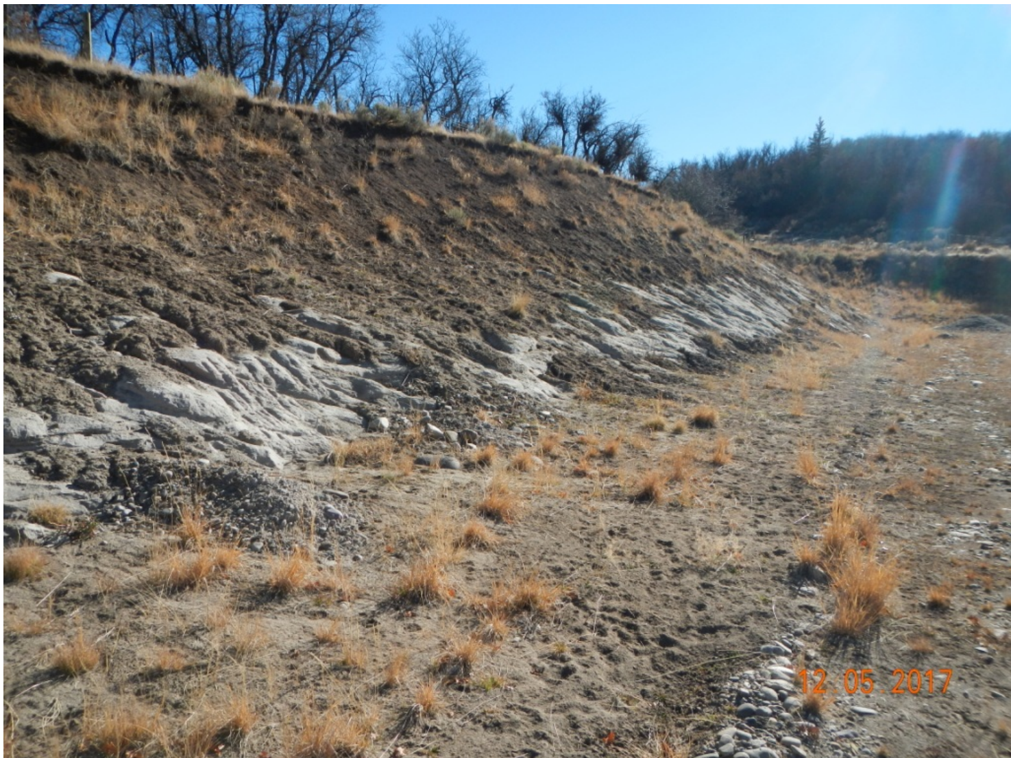
Photo 1. View of erosion occurring in the eastern portion of the project area. No stormwater controls have been installed.
