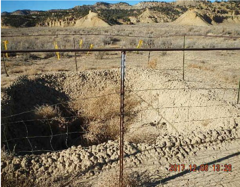
Blow down pit with animal burrow
