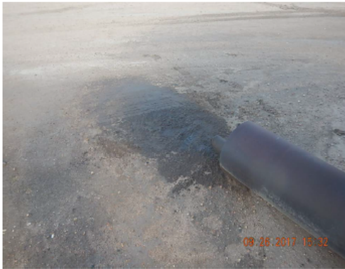
Photo 11: Stained soil at ajax exhaust
