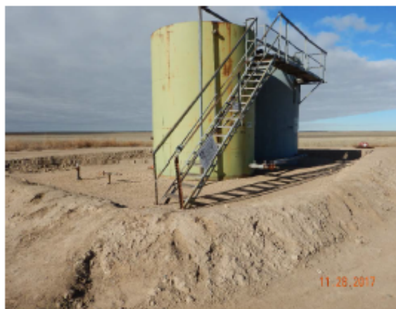
Photo #14 – View of crude oil tank battery from southeast corner. Note erosion of earthen berm and two (2) 2" steel flowline risers SW of tanks.
