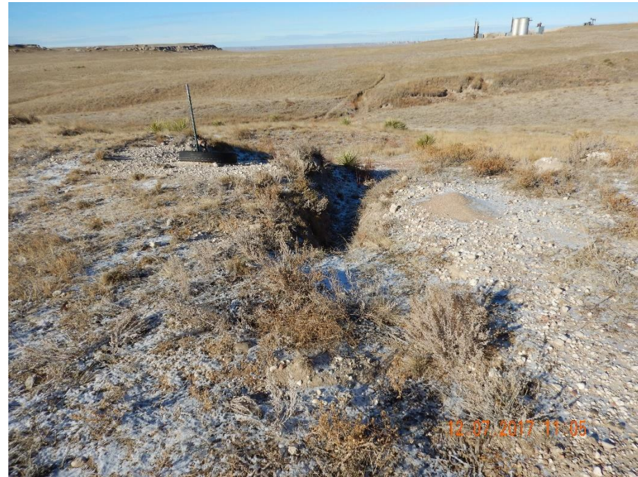
Photo 6: Photo taken from the west end of the location, facing west. Photo shows areas of erosion degradation. Erosion has not been repaired or stabilized and no BMPs have been installed or maintained per corrective actions.
