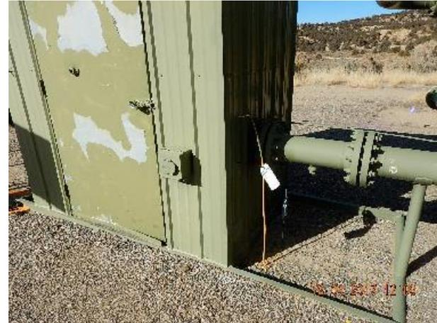
**Photo 12: Painted and tagged stainless steel line at gas meter house. Current inspection.**
