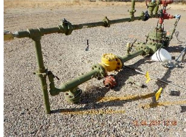
**Photo 6: Valve, nipple, and production related materials at wellhead. Current inspection.**
