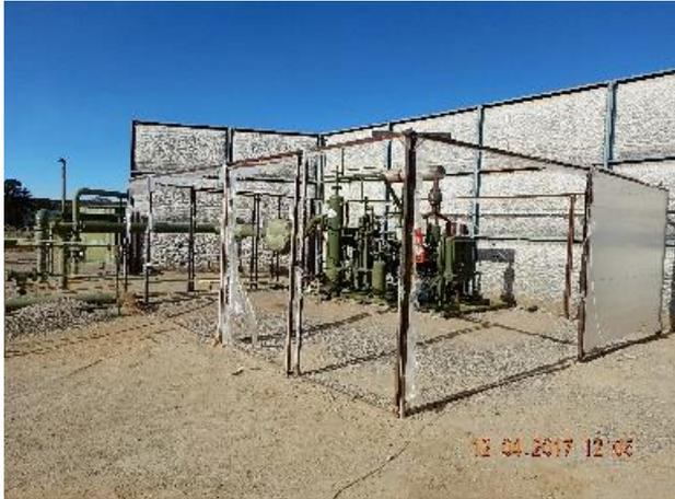
**Photo 11: Framing around compressor where plastic debris is tearing away from. Current inspection.**
