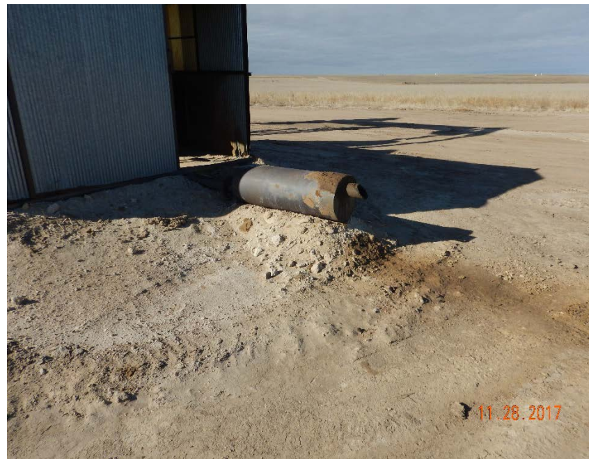
Photo #8 – Localized accumulation of oil-stained soil at prime mover exhaust.
