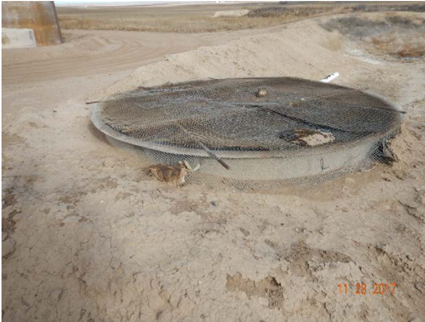
Photo #25 – View of open-top skim tank from SE corner. Note oily rag and small stockpile of oily waste at skim tank.
