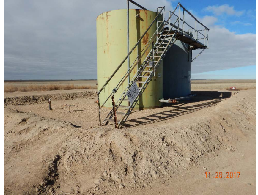
Photo #14 – View of crude oil tank battery from southeast corner. Note erosion of earthen berm and two (2) 2" steel flowline risers SW of tanks.
