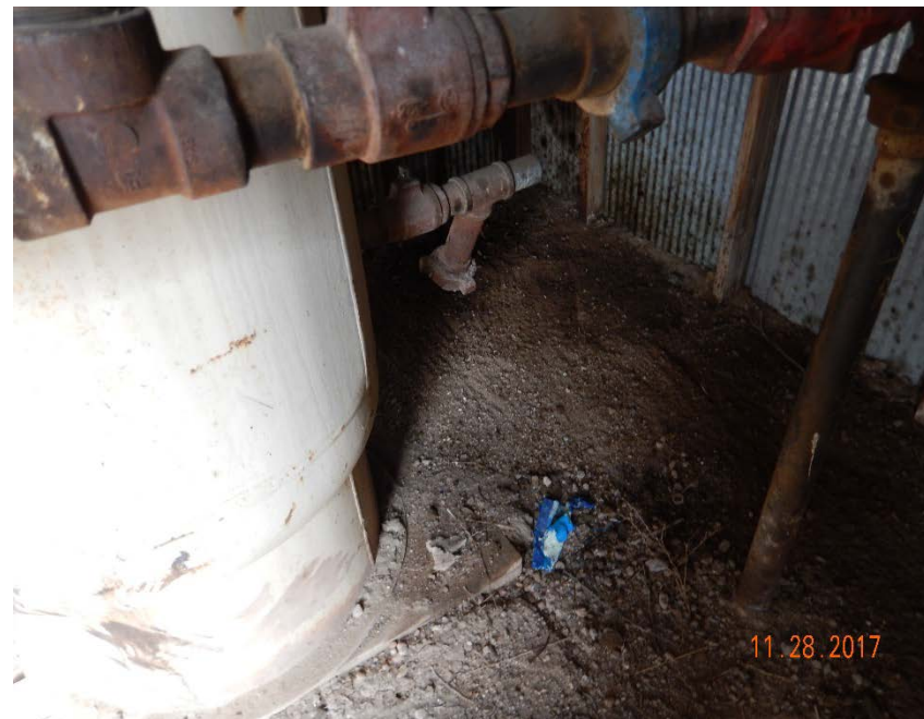
Photo #24 - Localized, oil-stained soil inside of separator/treater shed (3).
