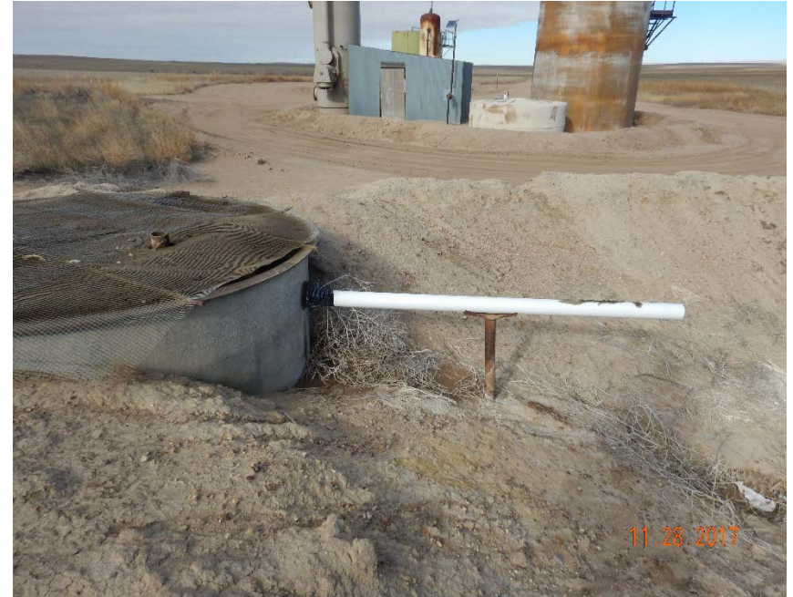
Photo #26 – View of skim tank outlet to south produced water pit. Note presence of oil-stained soil and weeds at tank outlet.
