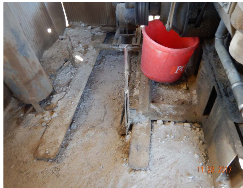
Photo #10 - Historical accumulation of oil-stained soil beneath prime mover (2).
