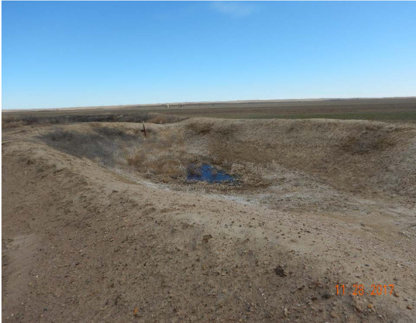
Photo #29 - NE portion of south produced water pit (Facility ID #273442). Note abundance of weeds and water present in pit.
