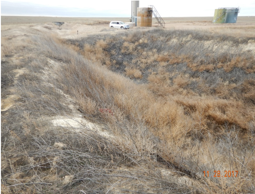
Photo #33 – Abundant weeds growing inside of berms of north produced water pit (Facility ID #273443), view from SE corner. Note oil-stained soil inside of berms in foreground.
