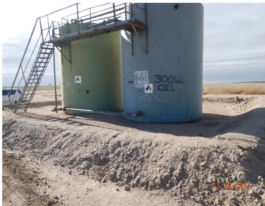
Photo #15 – Shallow, eroded tank berm at northeast corner.
