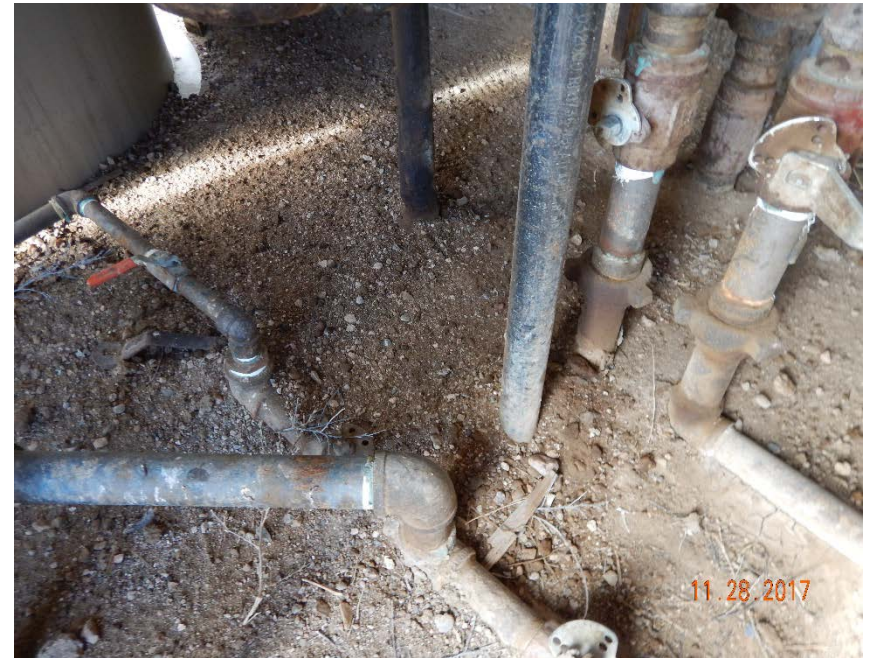
Photo #22 – Localized, oil-stained soil inside of separator/treater shed (1).
