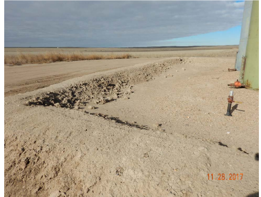
Photo #18 – Eroded earthen berm west of tanks.
