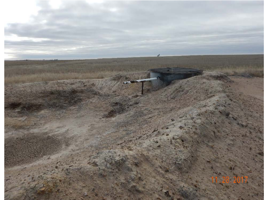
Photo #28 – SW portion of south produced water pit (Facility ID #273442). Note abundance of weeds and oil-stained soil.
