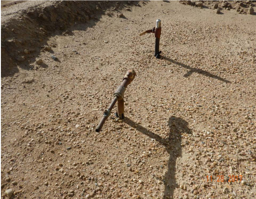
Photo #17 – Unused flowline risers SW of crude oil ASTs.
