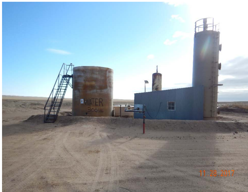
Photo #19 – View of 300 bbl produced water AST, produced water fiberglass PBV, and separator/treater shed from west side.
