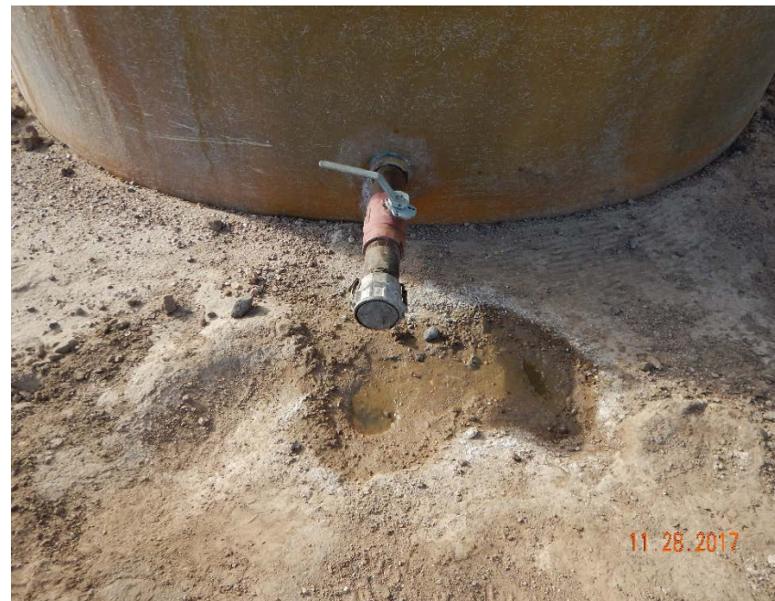
Photo #20 – Produced water pooling at fiberglass AST loadout valve.
