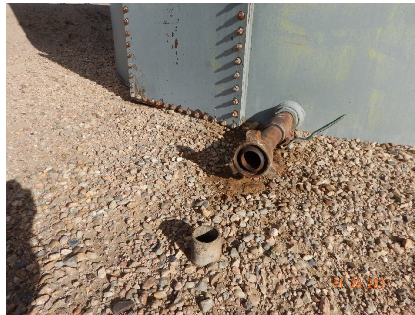
Photo #16 – Localized, oil-stained soil and uncapped pipe riser beneath tank valve.
