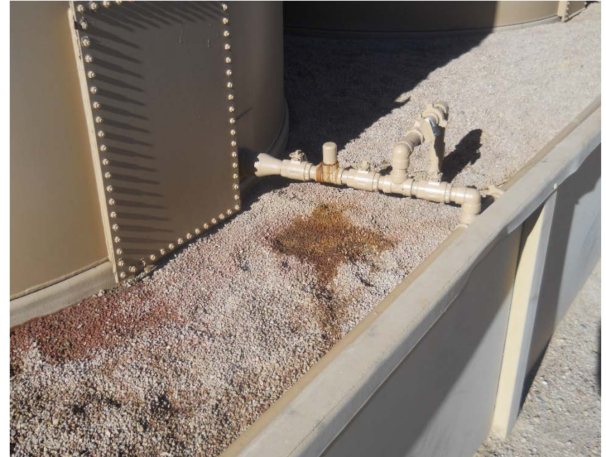
Stained soil at drain line on crude oil tank (11:32)
