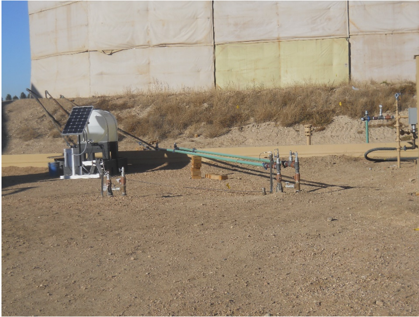
Hardline coming from Simpson FD 16-382HN wellhead west of separators (14:10)
