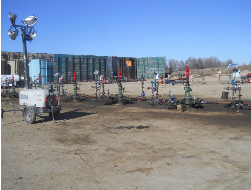
Wellheads looking northwest with flares northwest of them. Stained soil around wellheads (10:44)
