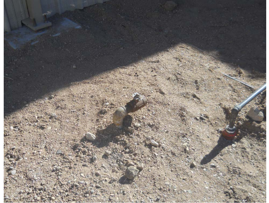
(#2)Unused/unmarked 2" steel riser at compressors (11:15)
