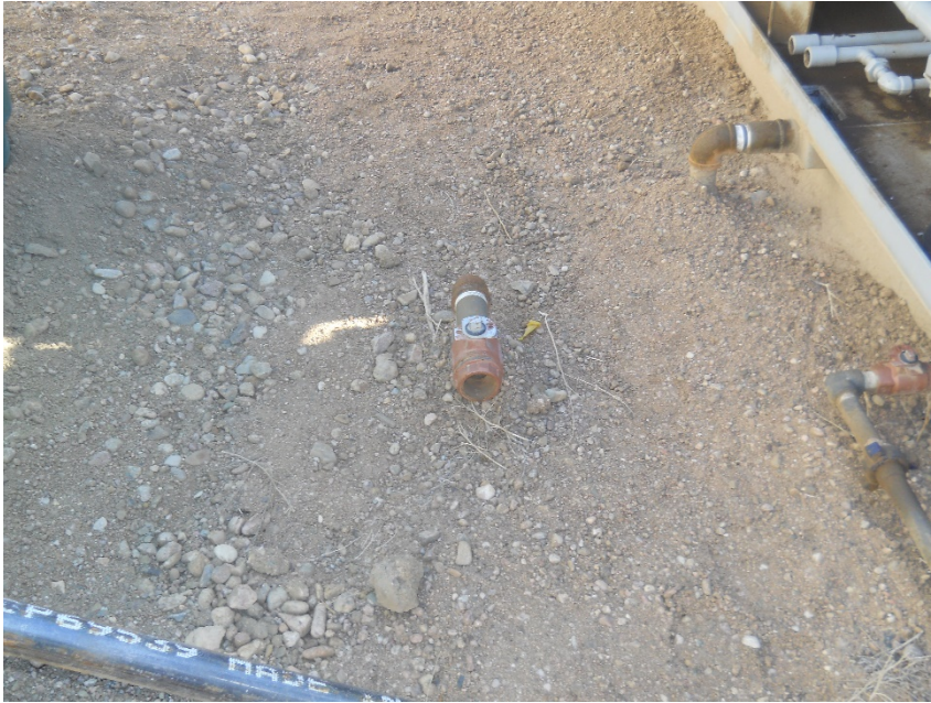
(#3)Unused/unmarked steel riser at compressors (11:17)
