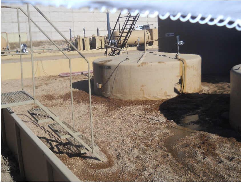
Stained soil around north production water tank (11:35)
