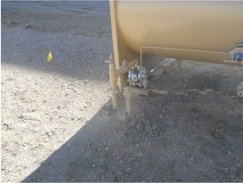
1" unused/unmarked steel riser at ECD knockout (11:32)
