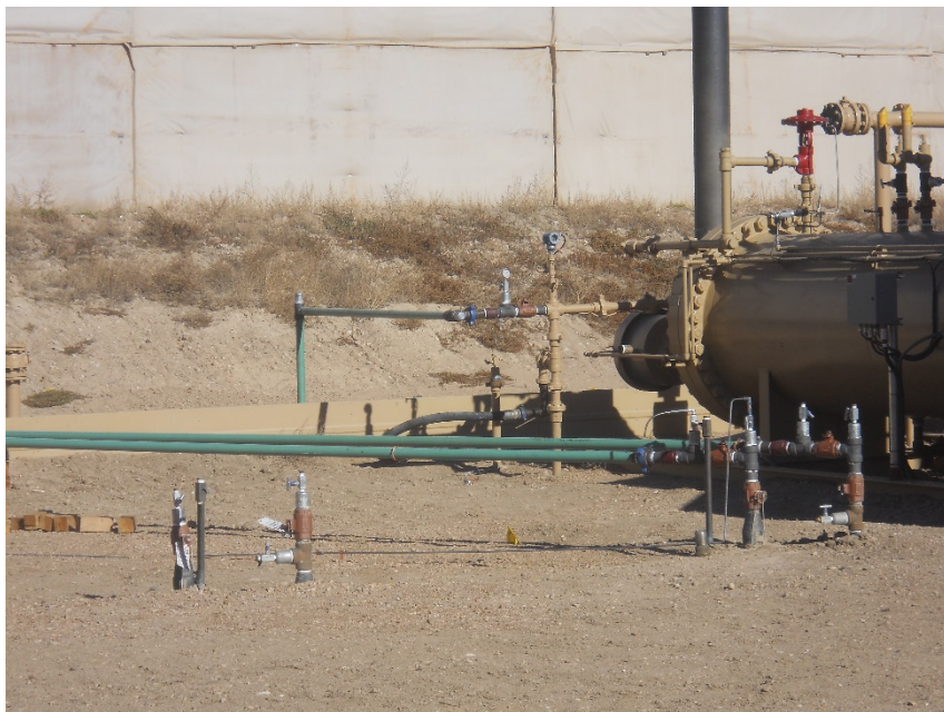
2-1" unused/unmarked steel risers, 1-2" unused/unmarked steel riser, 2-2" marked/unused steel risers west of separators (11:24)
