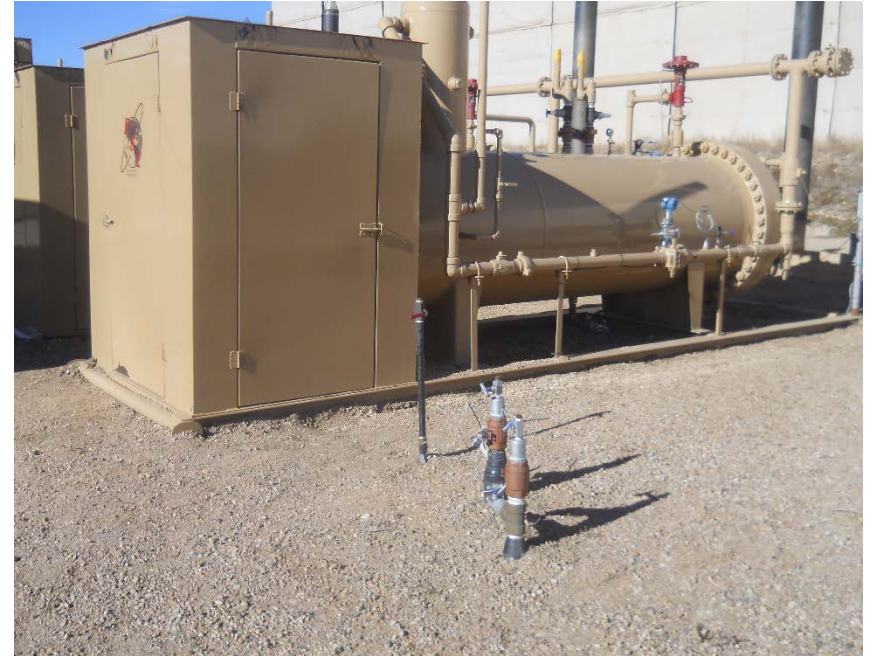
1" unused/unmarked steel riser and 2-2" steel marked/unused risers east of separators (11:20)
