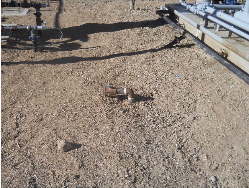
(#1)Unused/unmarked 2" steel riser at compressors (11:15)
