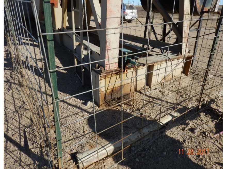
Photo #4 – Localized, oil-stained soil beneath SW corner of pump jack.
