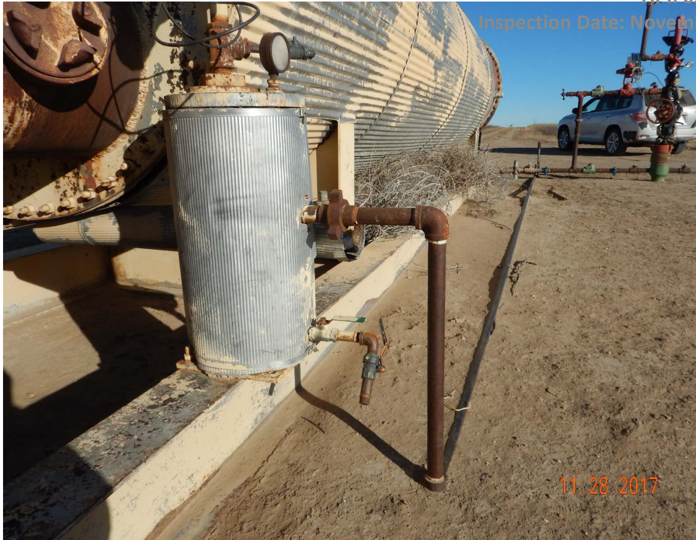
Photo #3 – 1" flowline riser and accumulation of wind-blown weeds on east side of separator.
