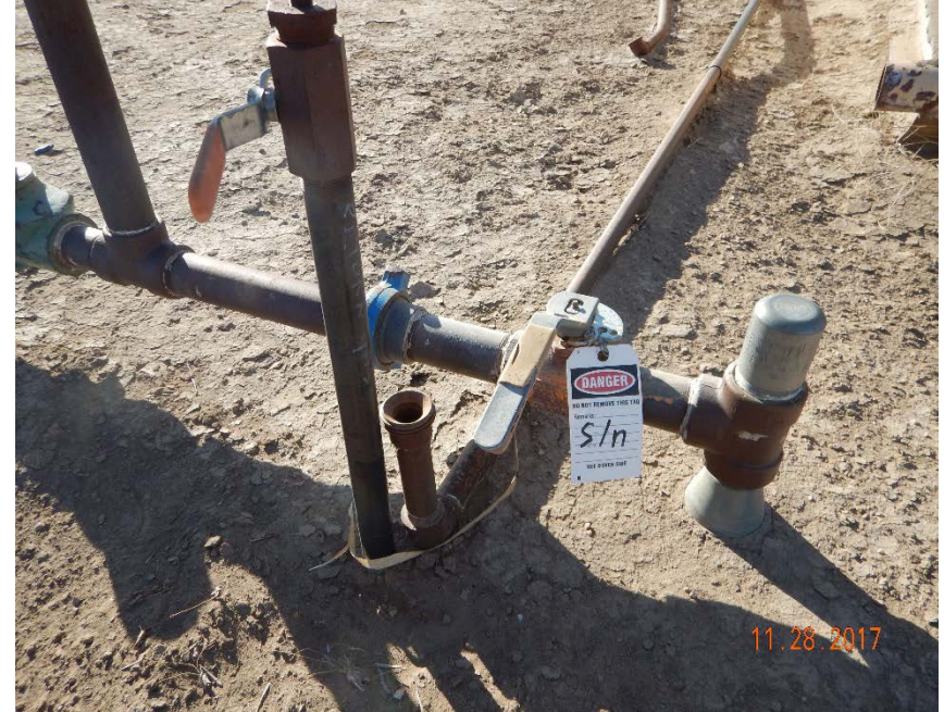
Photo #2 – Uncapped, 1" flowline riser leading from separator to wellhead alongside tagged-out and bullplugged 2" riser west of wellhead.
