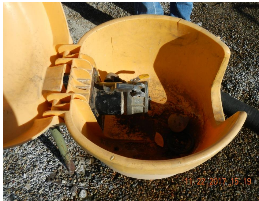
Cap on load out line was tightened by XTO representative during inspection of facility.
