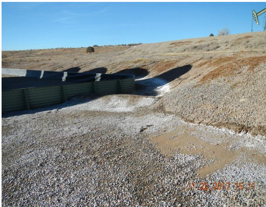
Damp soil and white residue in northwest corner of tank battery.
