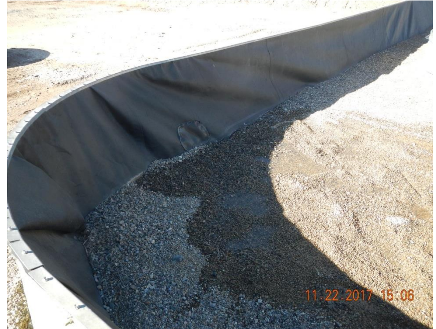
Patched liner in SW corner of containment area.
