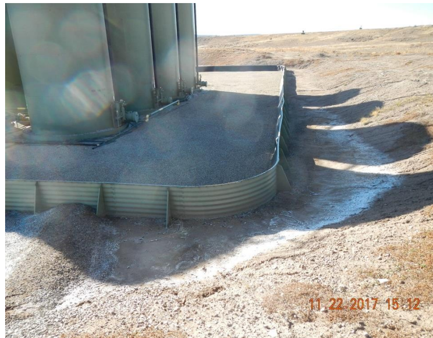
White residue and damp areas on north and east side of tank battery.
