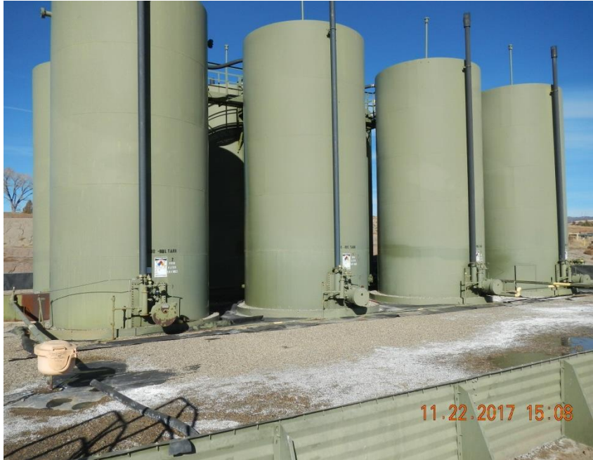
Standing water and white residue inside secondary containment area.
