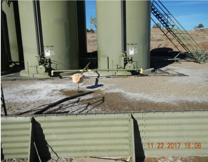
Load out valve was leaking upon arrival. Drip pot is cracked and not functioning properly.
