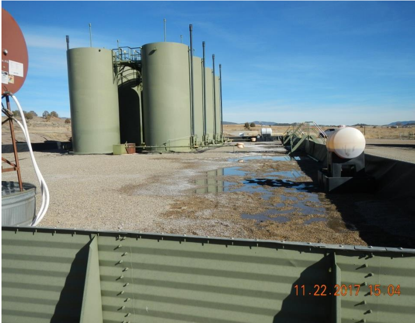
Standing water in secondary containment area.
