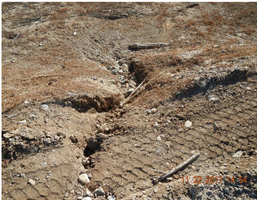
Erosional channel forming along southern edge of pad.
