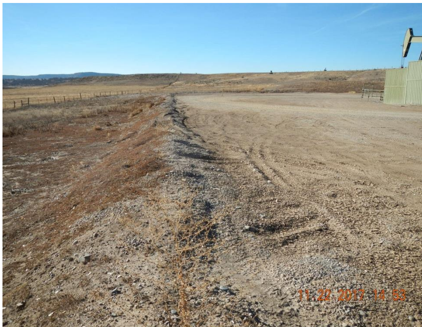
Location berm along southern edge of pad.
