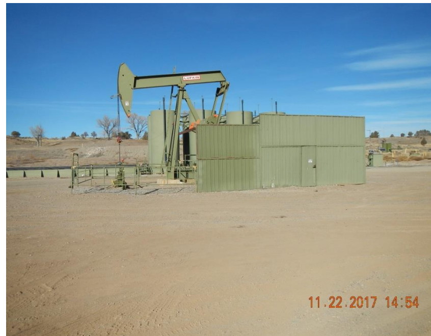
Hein #1-2 pump jack and well head. Tiffany Lease Tank Battery in the background.
