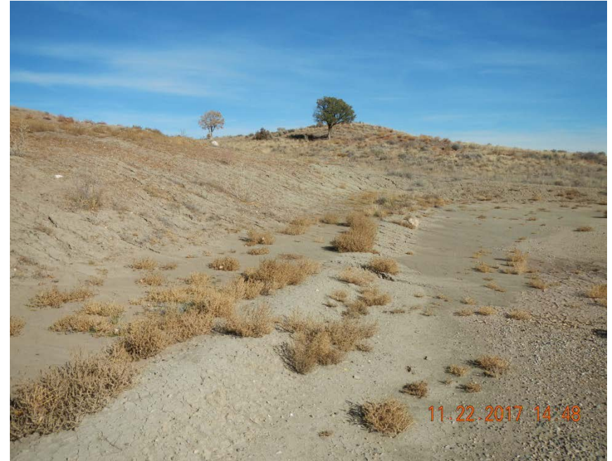
Run on control berm has filled in with sediment.
