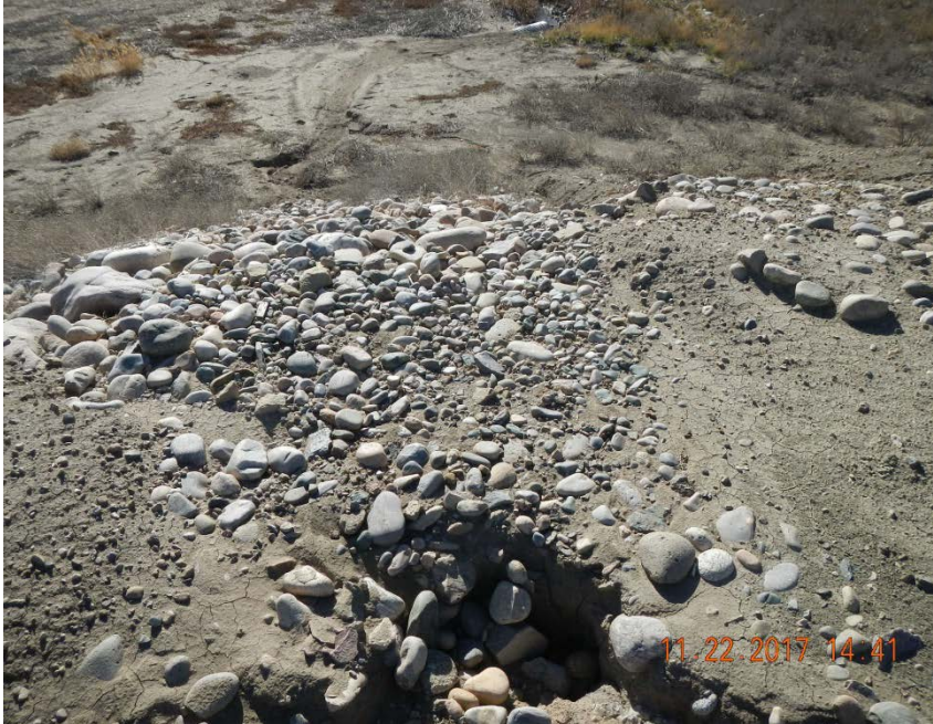
Rip rap run down in SW corner of location requires maintenance.
