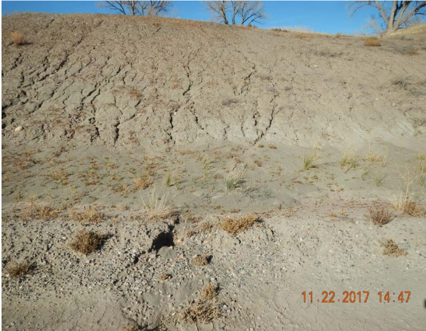
Location berm has been breached.
