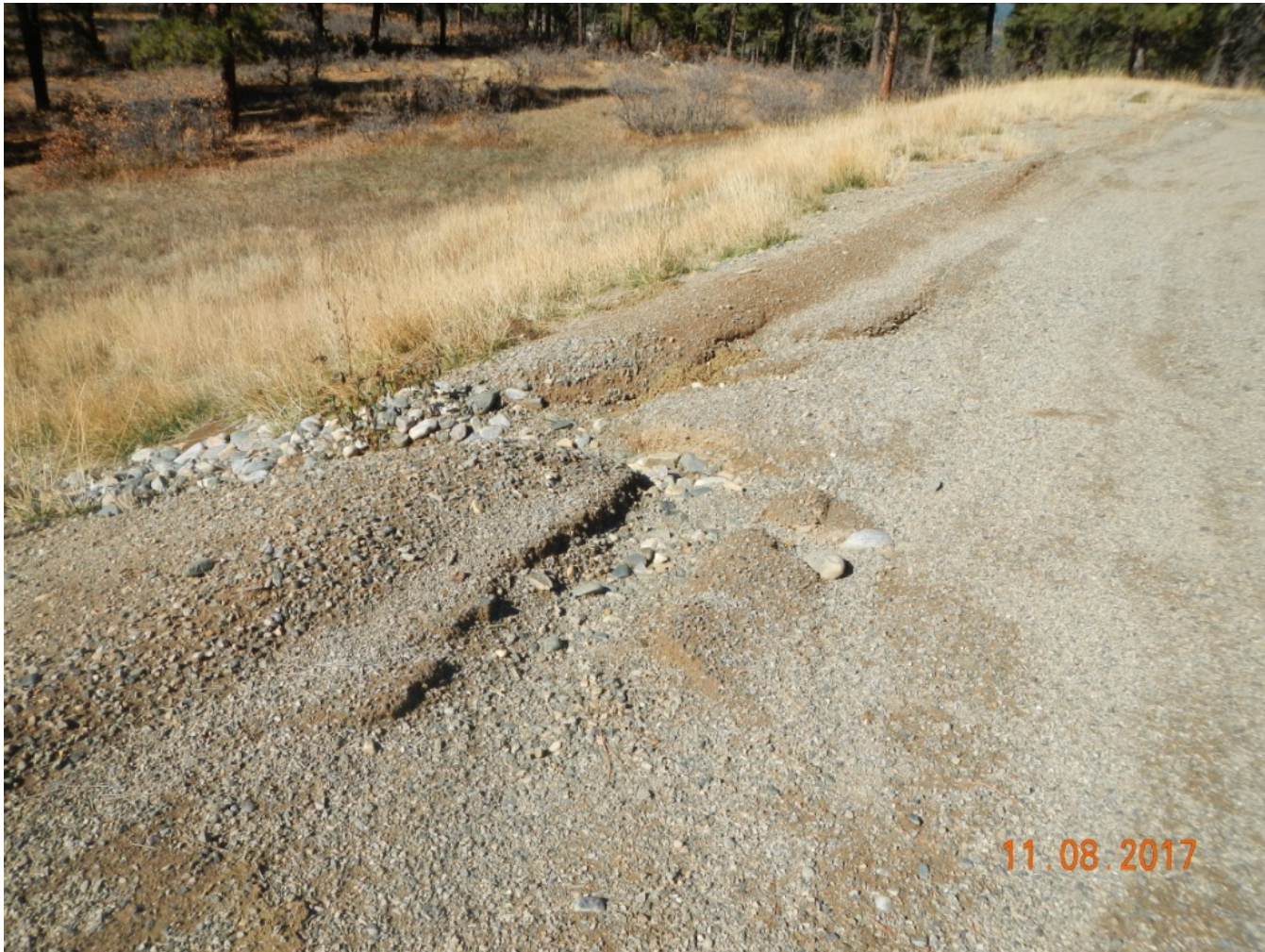
Photo 5. View of area in the western project area where concentrated flows are eroding and stormwater controls need maintenance.
