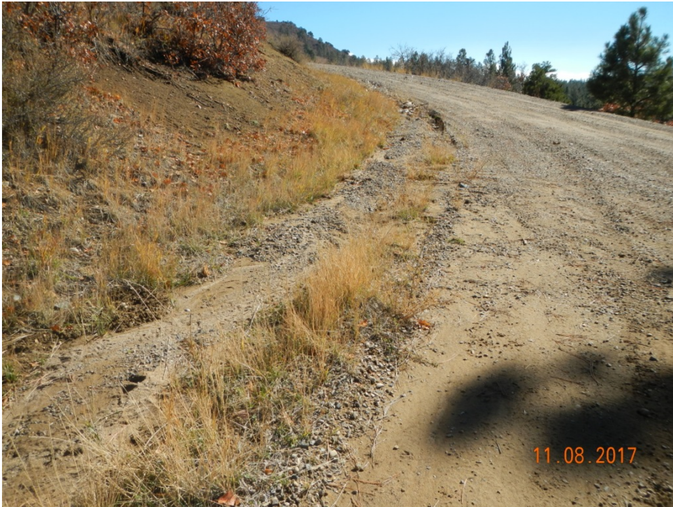
Photo 4. View of the erosion occurring at the access road entrance. Ditch is full of sediment and stormwater is diverted and flows across lease road.
