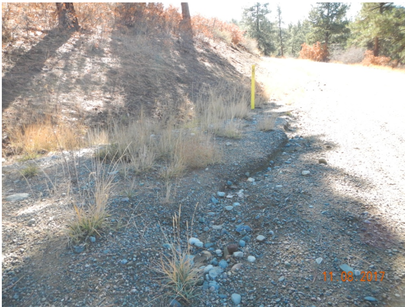
Photo 6. View of erosional channel forming at the well pad entrance where diverted stormwater flows off of the eastern well pad.
