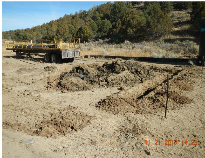
Containment trench dug around stained soil.
