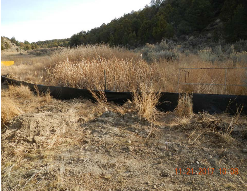
Silt fence installed by A+ Well Services.
