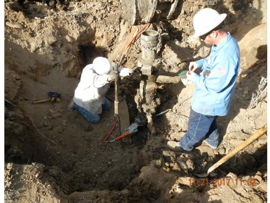
Cutting off wellhead.
