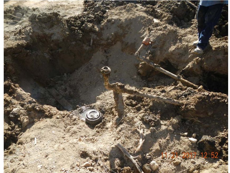
Flowline terminations near cut off well head.
