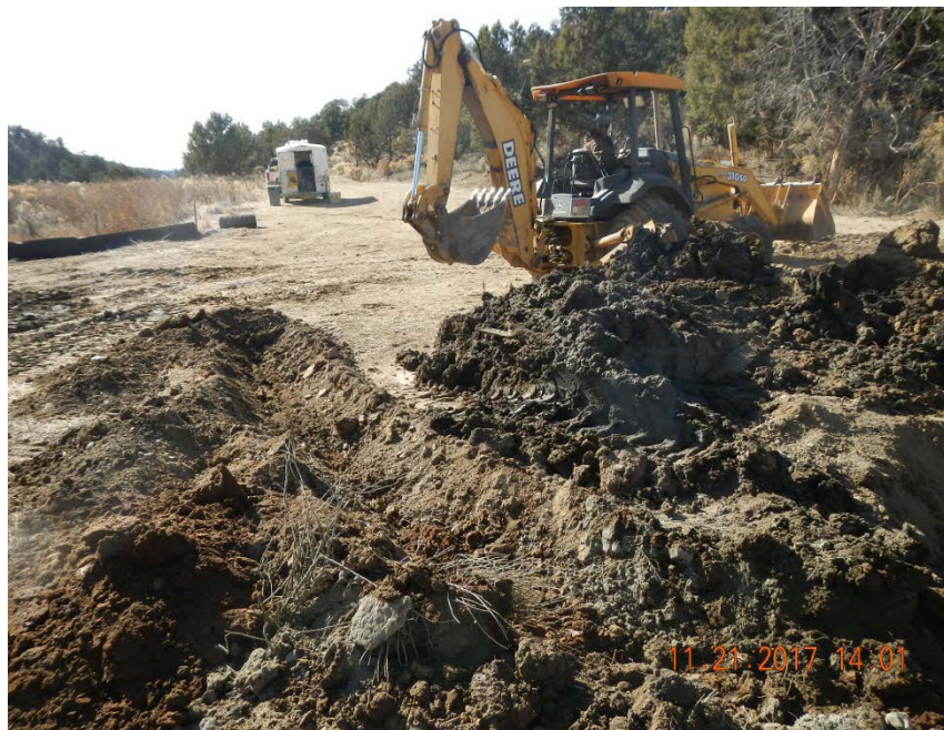
Back hoe digging perimeter trench around impacted material.
