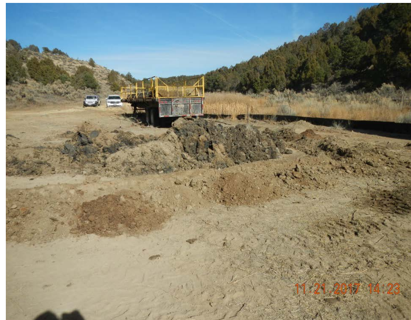
Photo of containment trench on downhill sides of stain soil stockpile.
