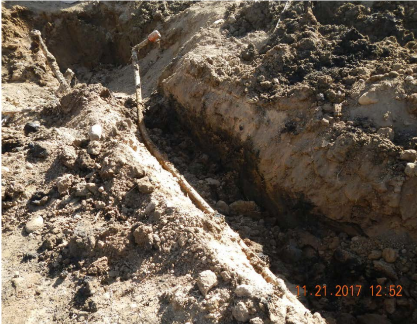
Impacted material surrounding flow lines.
