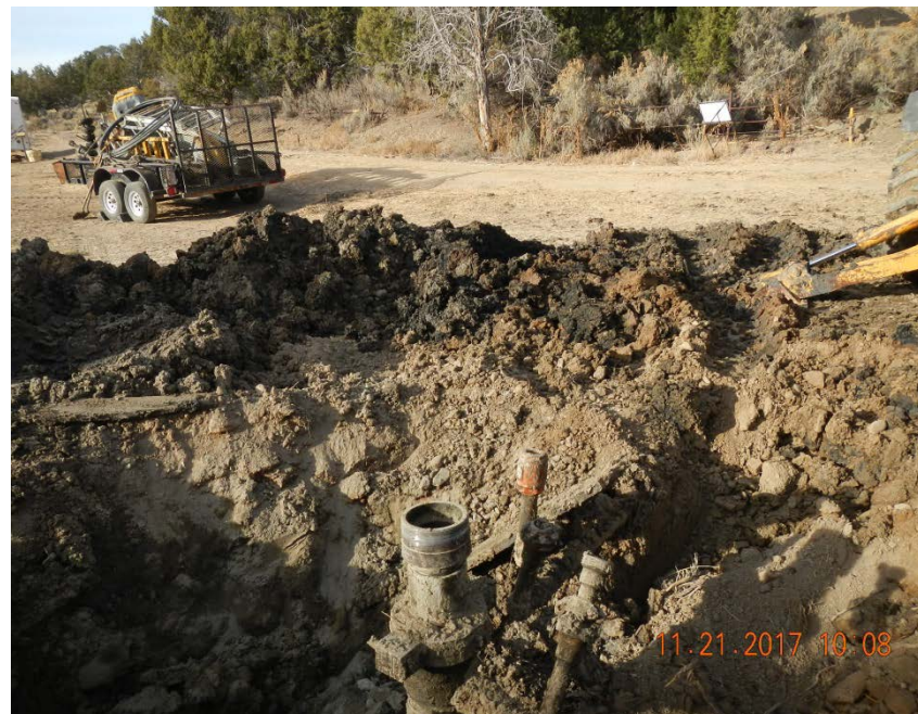
Impacted material excavated from around wellhead.
