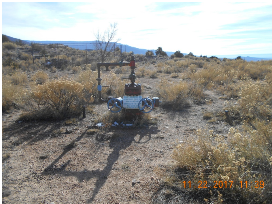
Location 05-077-08264. Capped risers near wellhead.
