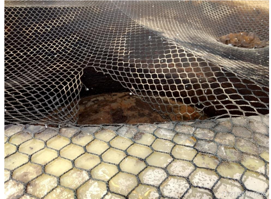
Produced water tank detail, Corrective Action: Netting on open tanks inadequate. Wildlife protections devices not adequate.
