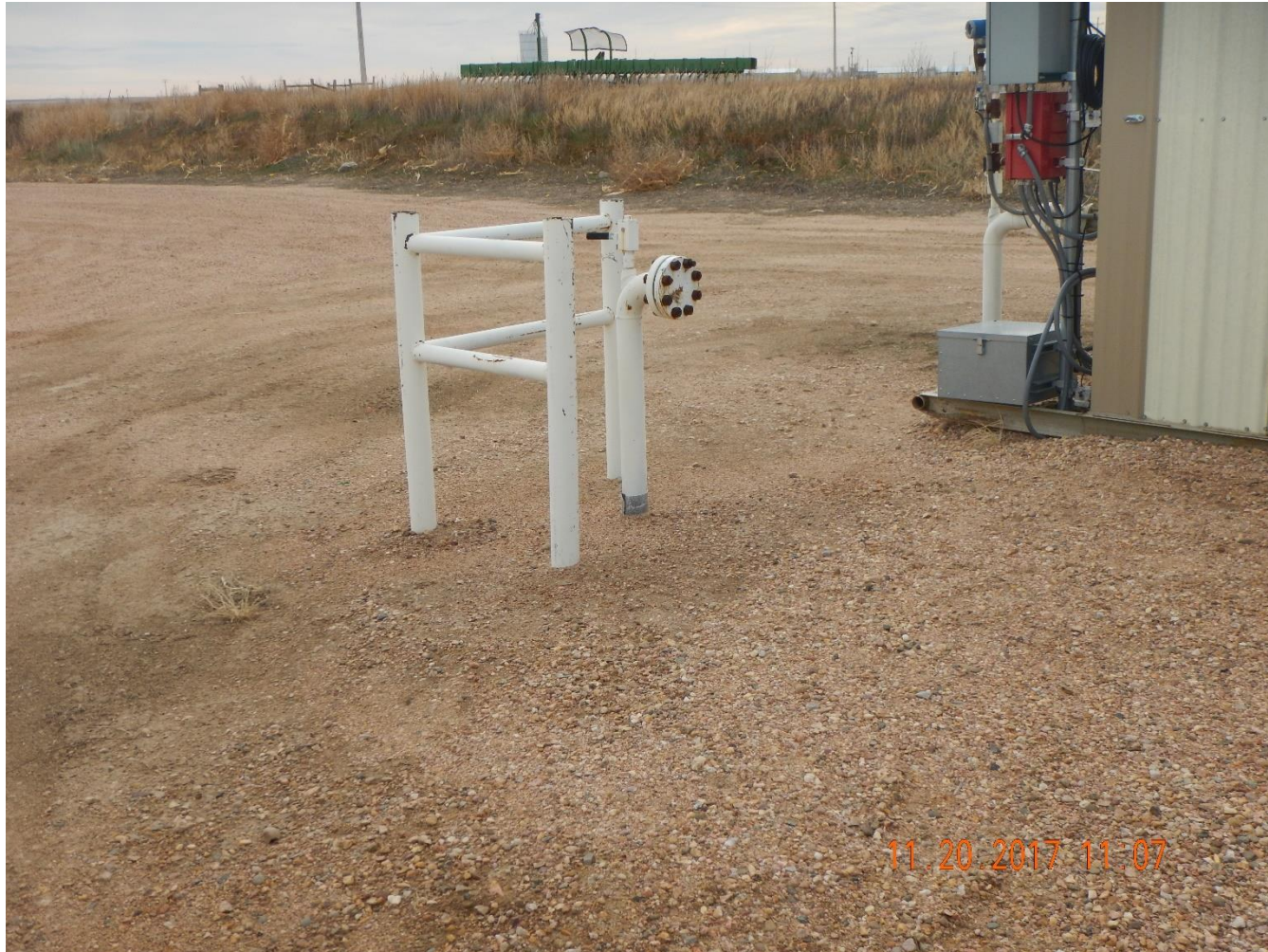
Photo 1: Photo taken from the west end of battery location. Inspection #682502655 required operator to remove riser. Photo shows riser has not been removed per 1004.a
