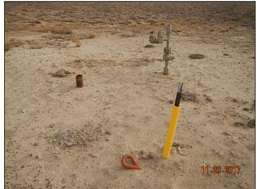
Photo 2. Unmarked riser.
