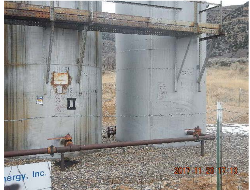
Tank 3 missing NFPA placard
