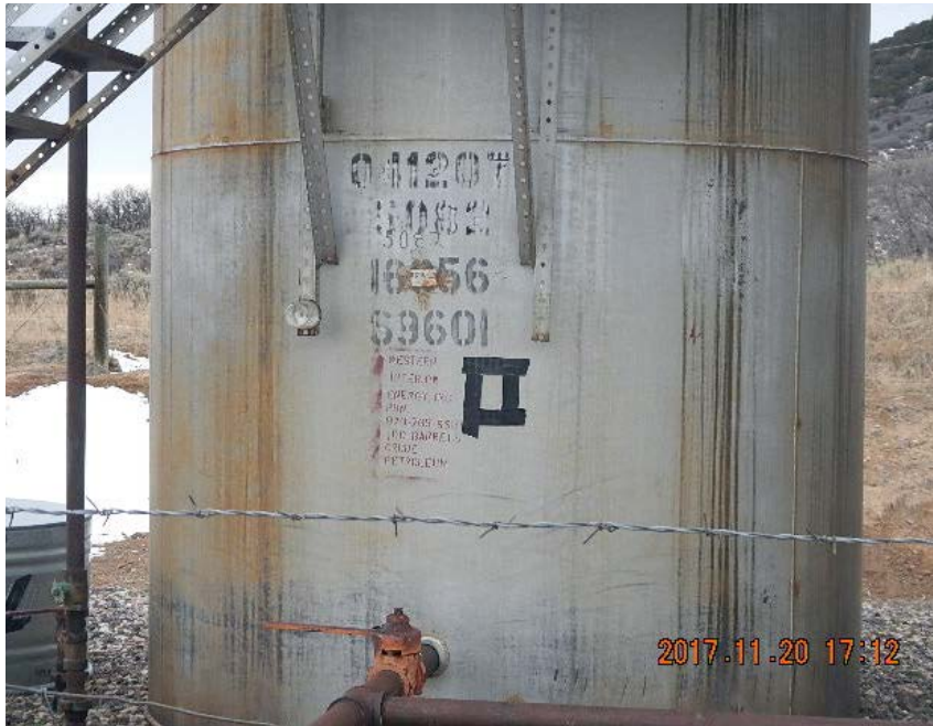
Tank 1 – missing NFPA placard
