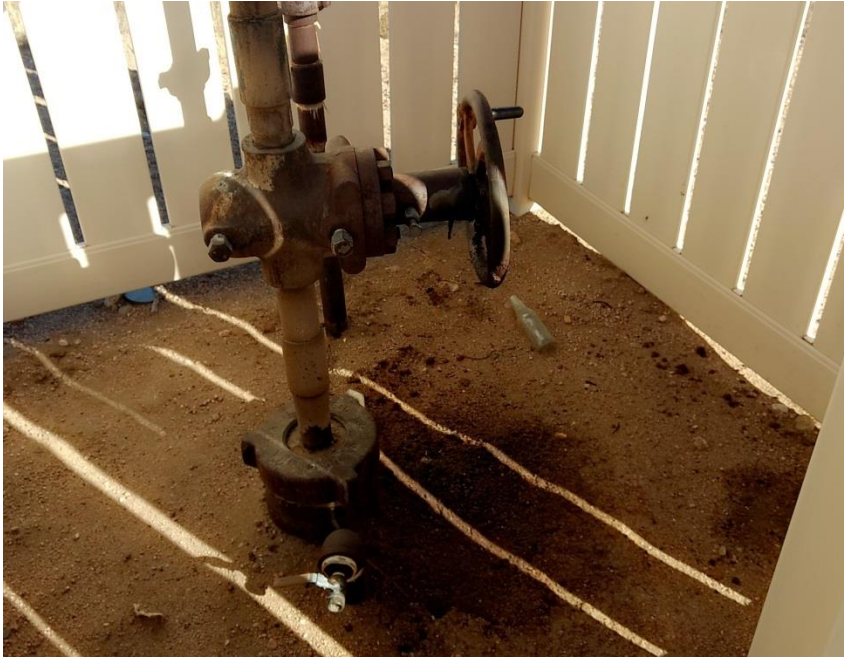
Wellhead, Corrective Action: Packing in master valve appears to be leaking causing stained soil.
