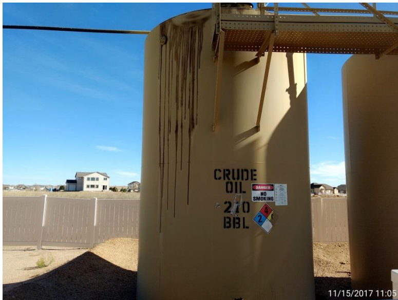
North Production Tank Detail, Corrective Action: Staining on Side of Tank.
