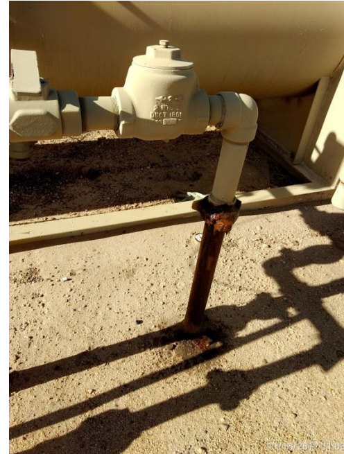
Riser at Separator Detail, Corrective Action: Leaking Hammer Union, Stained Soil.
