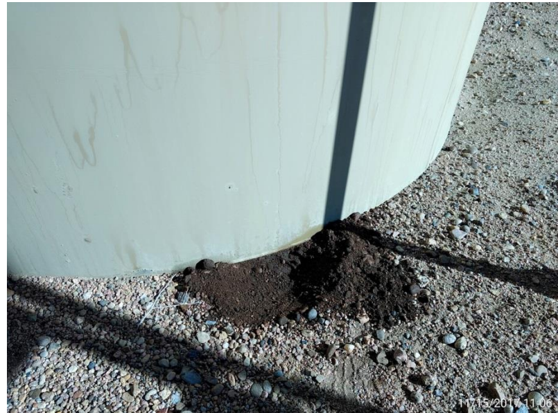
South Production Tank Detail, Corrective Action: Stained soil at base.
