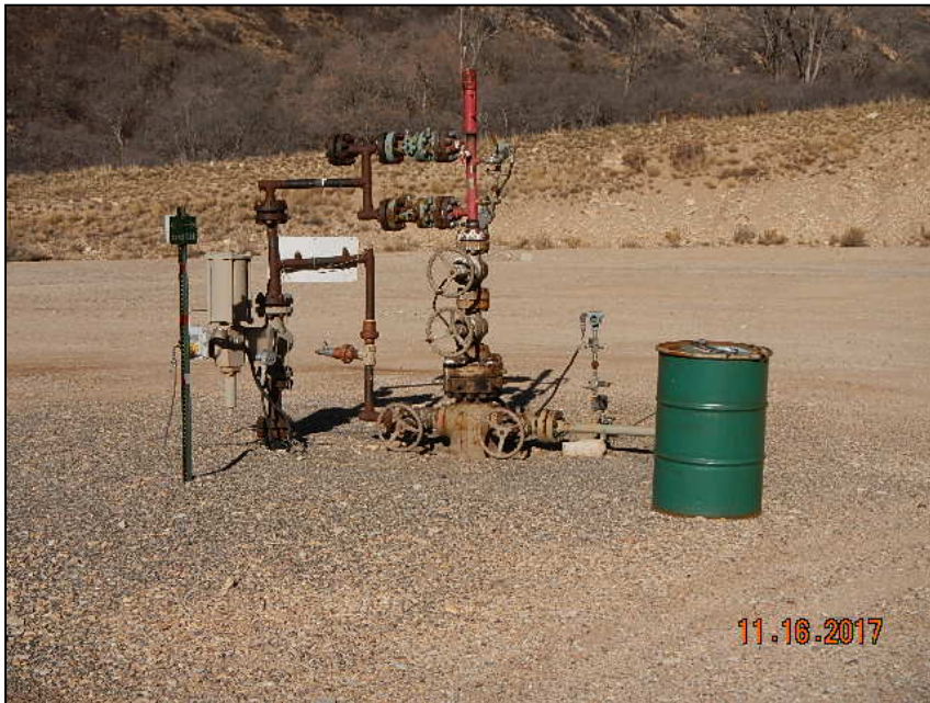
Photo 1. Barrel at wellhead w/ no containment.
