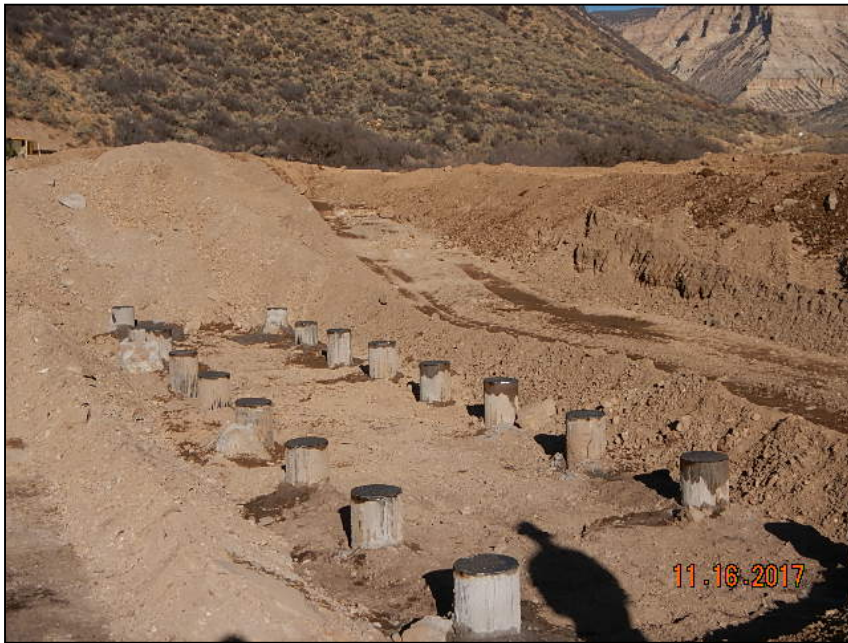
Photo 1. Wellheads. Plugged and cut off.
