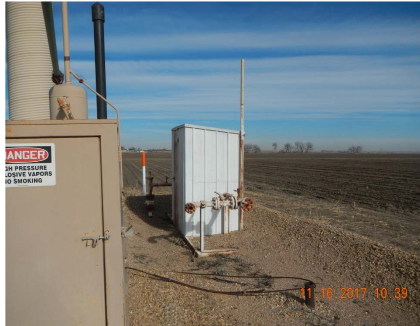
Unused meter run and pig station
