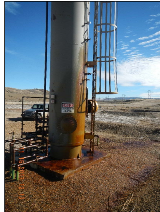
Photo 6. Broken sight glass on separator and fluid in separator berm.
