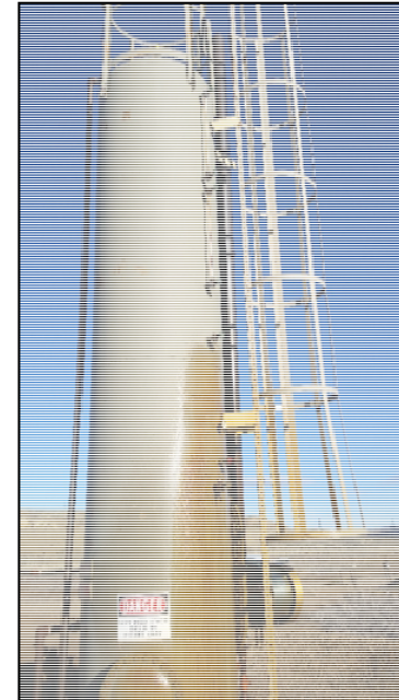
Photo 2. Broken sight glass on separator.
