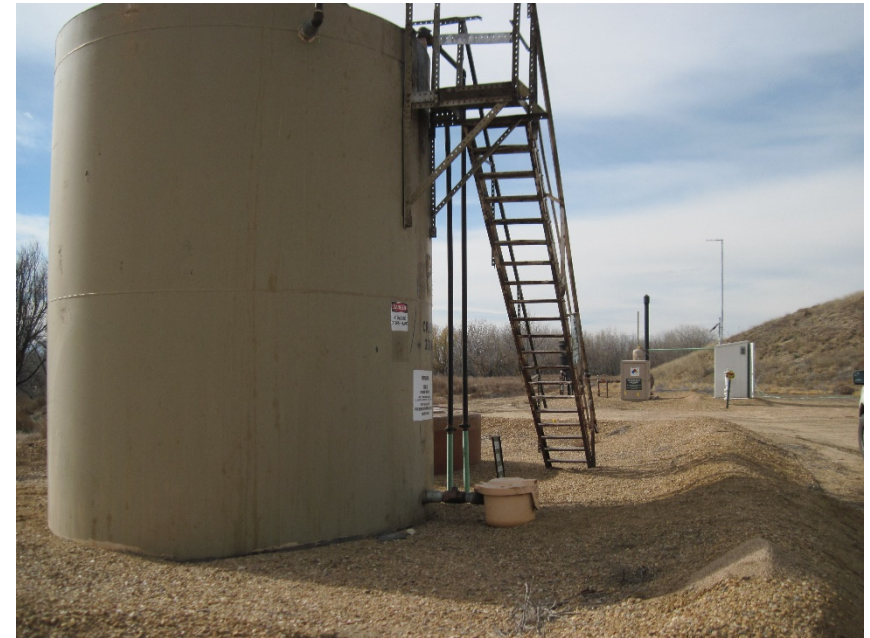
Tank battery and prod equipment no tie downs on separator, oil prod tank, water tank
