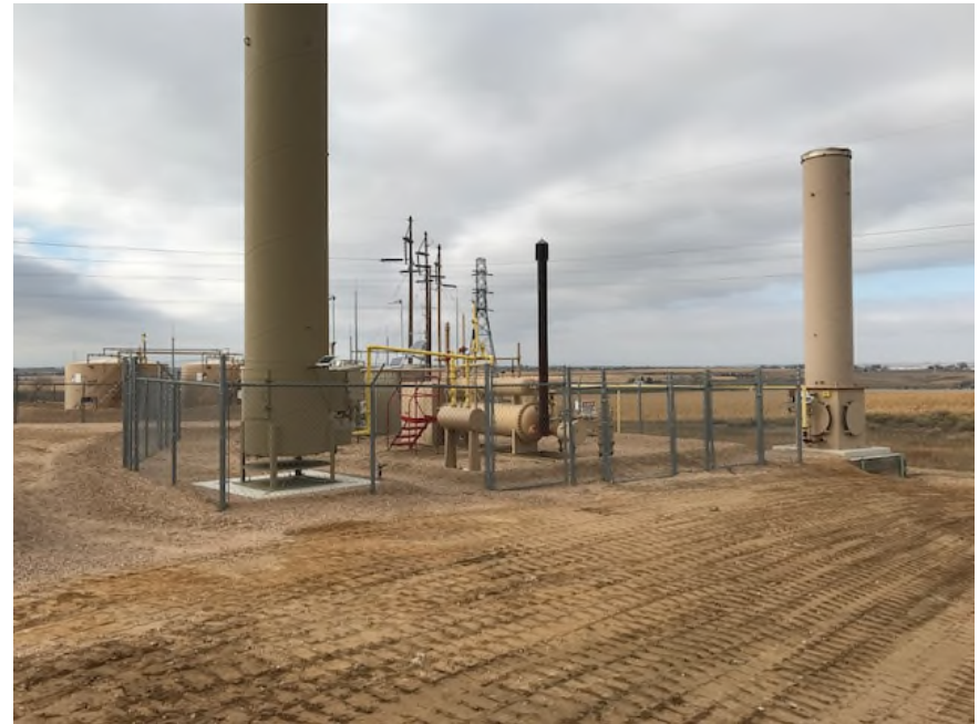
Photo NBL2. Repaired areas of erosion and tracked the slope of the pad.
