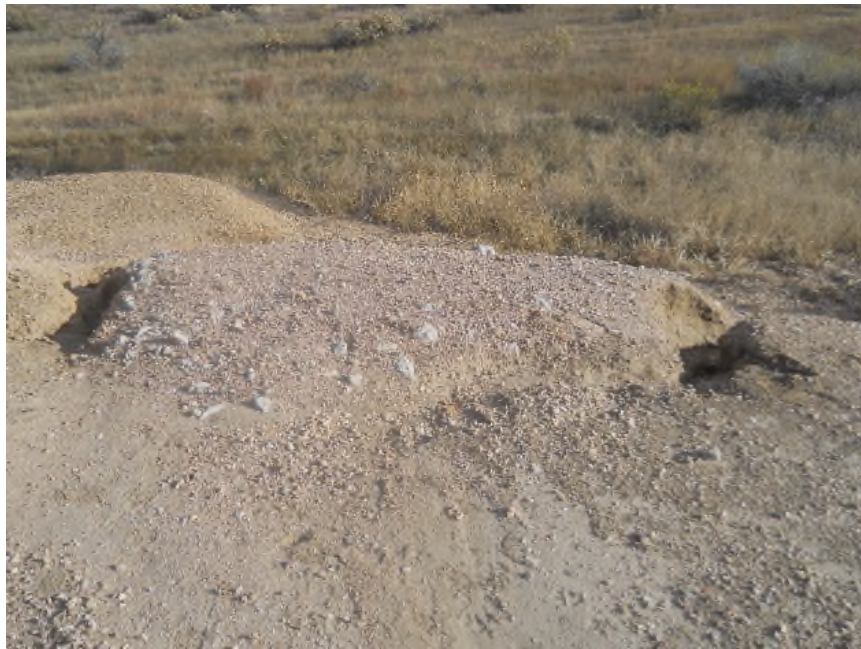
Photo 1. Location is washing out on east side of location, discharging sediment off of location.
