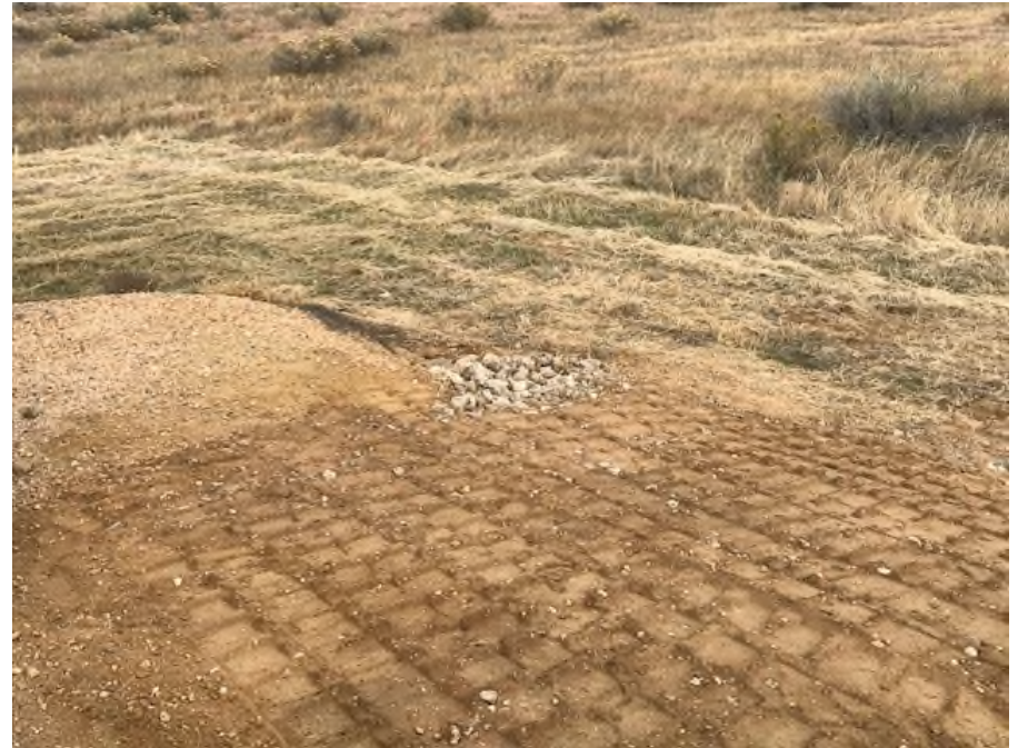
Photo NBL1. Repaired areas of erosion and installed larger rock at the discharge point.
