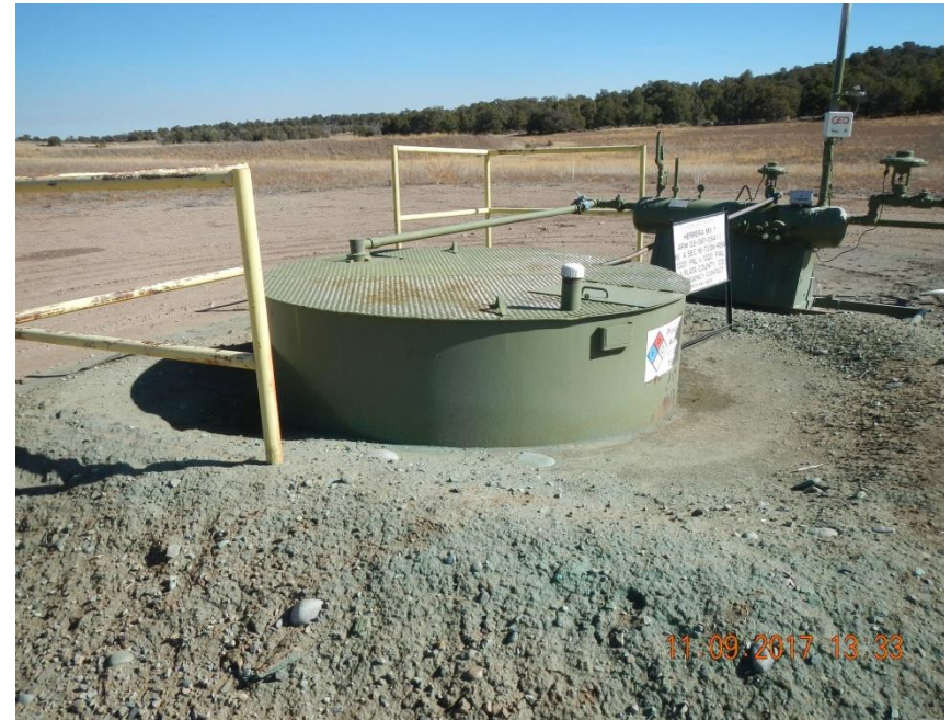
Produced water vessel with insufficient capacity of secondary containment.
