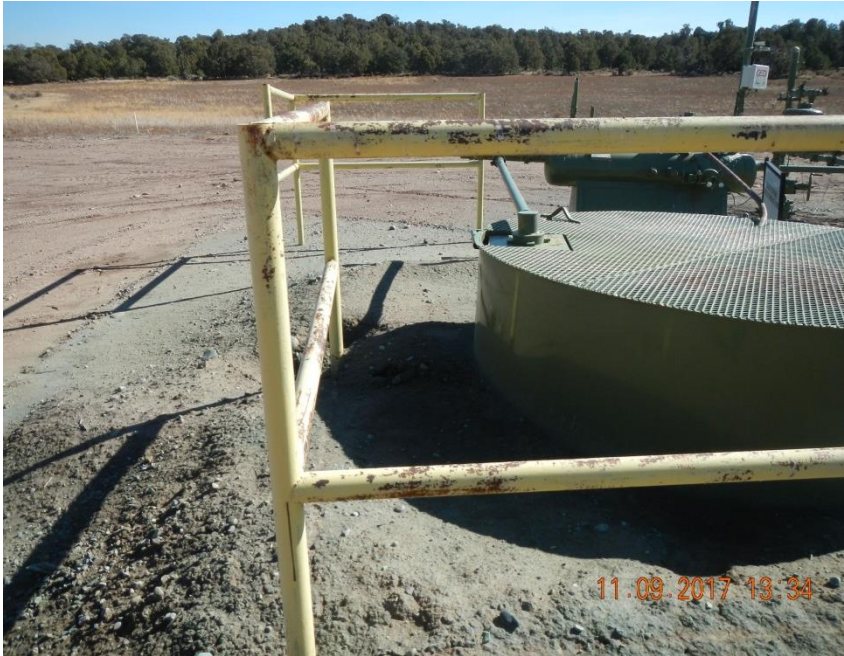
Secondary containment berm with insufficient capacity.
