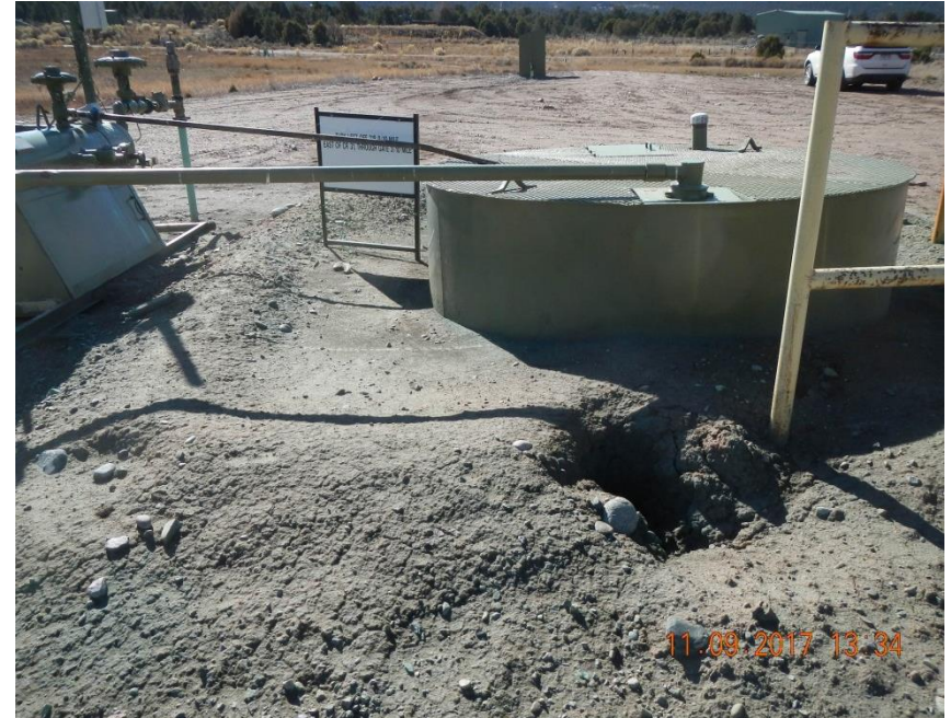
Animal burrow further compromising secondary containment berm.
