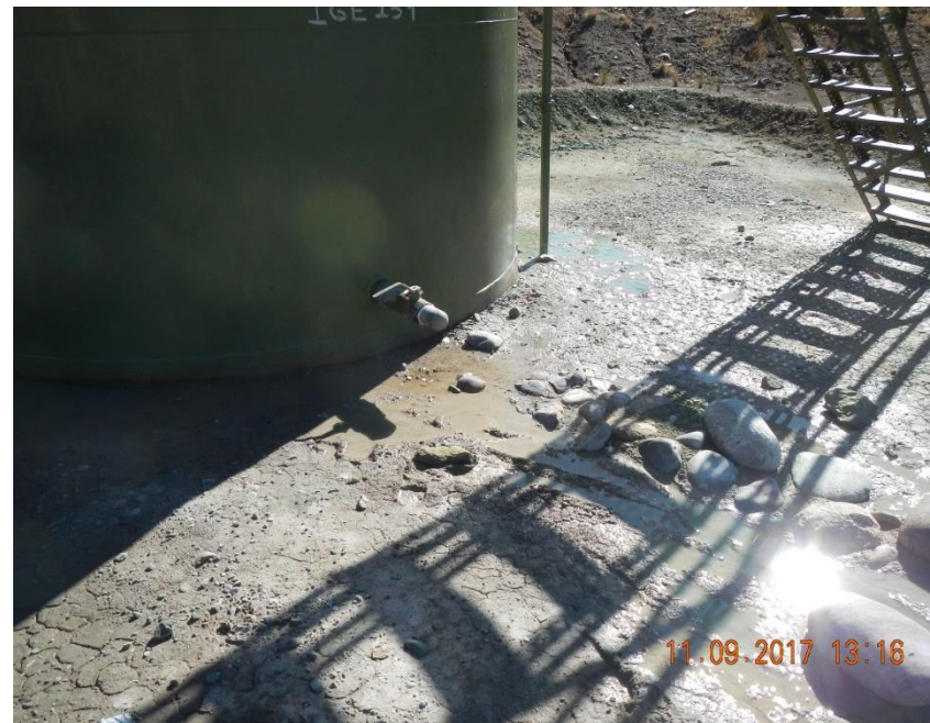
Load out valve leaking during field inspection.
