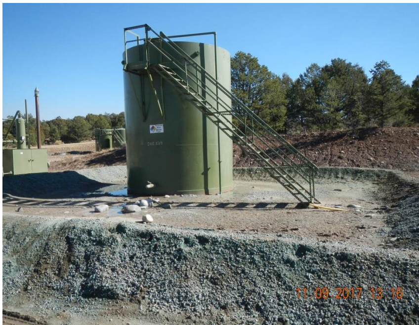
300 bbl. PW AST with earthen berm.
