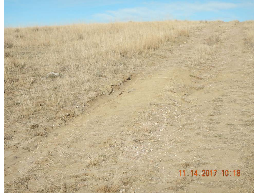
Photo 2: Stormwater erosion along access road
