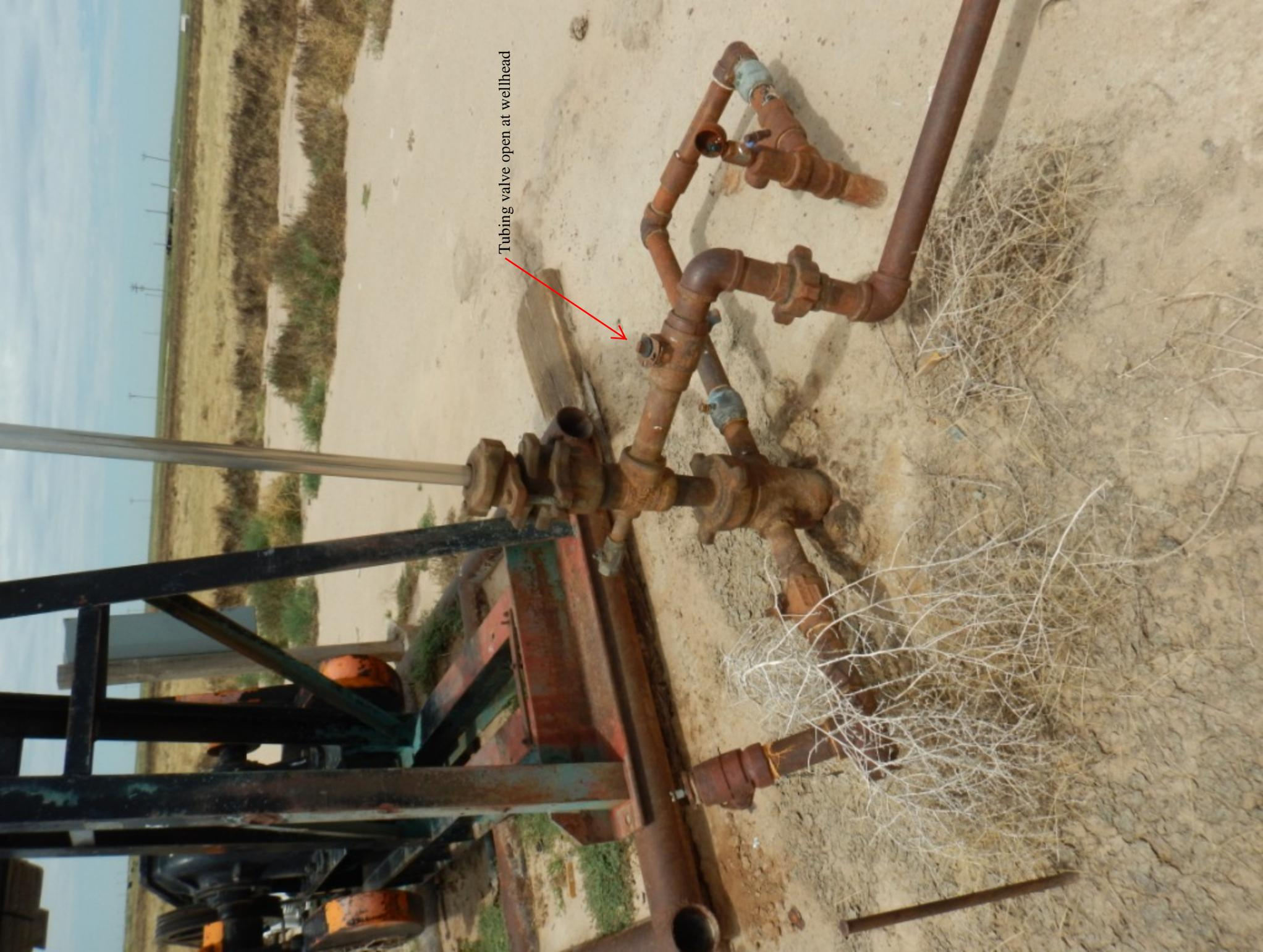
Tubing valve open at wellhead
