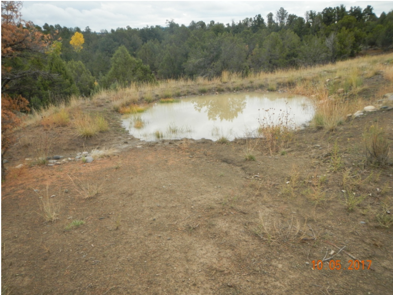
Photo 4. View of silt trap in the northeastern portion of the project area. Evidence of overflow and erosion downstream indicates silt trap needs maintenance.
