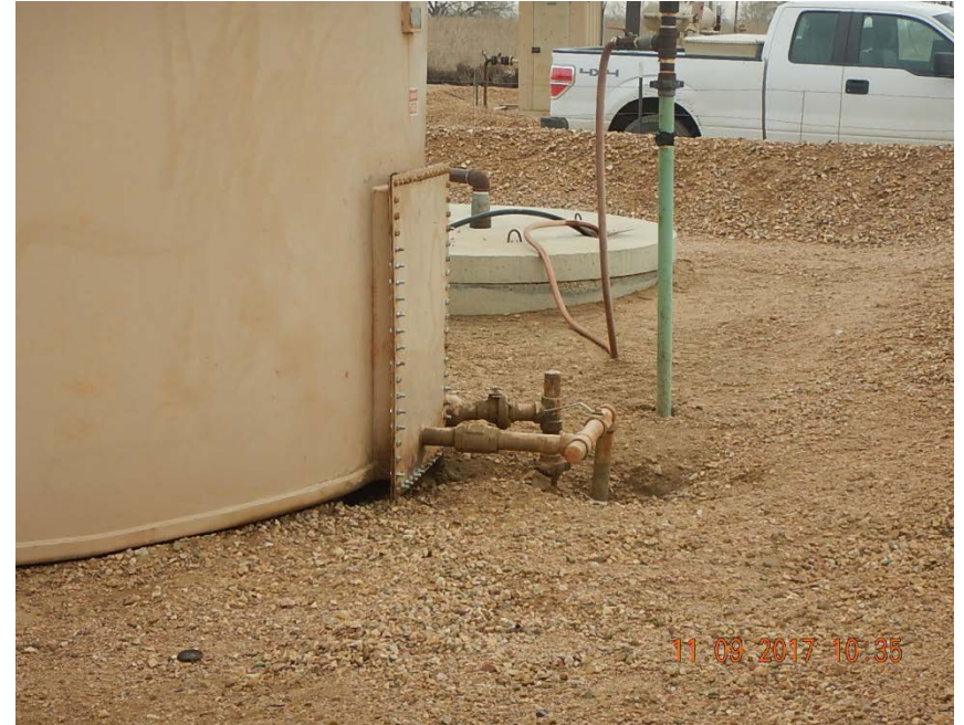
Photo 4: Leak repaired, stained soil removed
