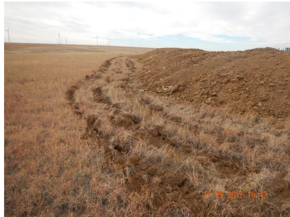
Photo 2: Photo taken from the southeast end of the location, facing west. Operator installed surface roughening as a stormwater and sediment control BMP around the perimeter of the location. BMP had been installed prior to construction activities.
