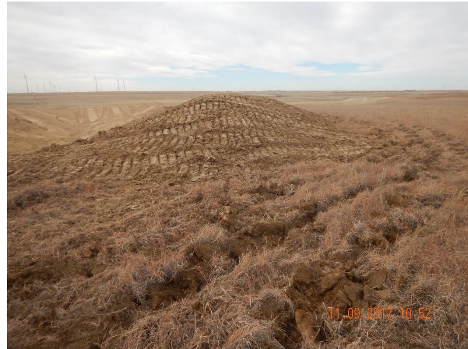
Photo 4: Photo taken from the north end of the location, facing west. Photo shows topsoil salvage and stabilization in process.
