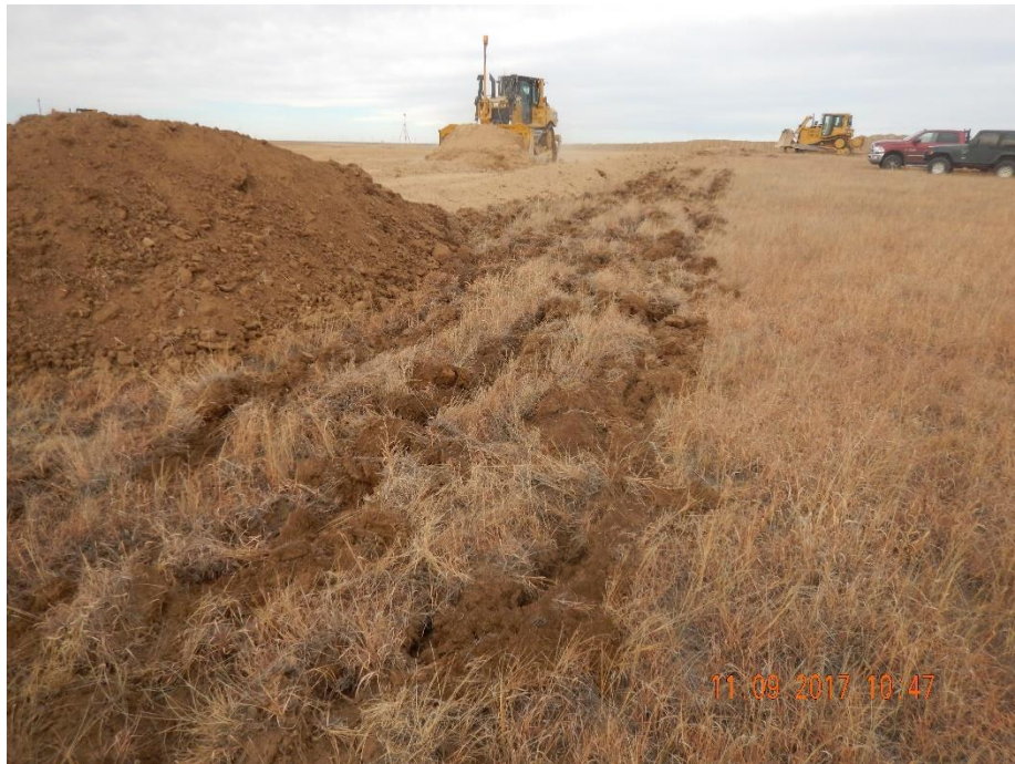
Photo 1: Photo taken from the southeast end of the location, facing north. Operator installed surface roughening as a stormwater and sediment control BMP around the perimeter of the location. BMP had been installed prior to construction activities.
