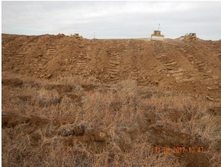
Photo 3: Photo taken from the north end of the location. Photo shows topsoil salvage and stabilization in process.
