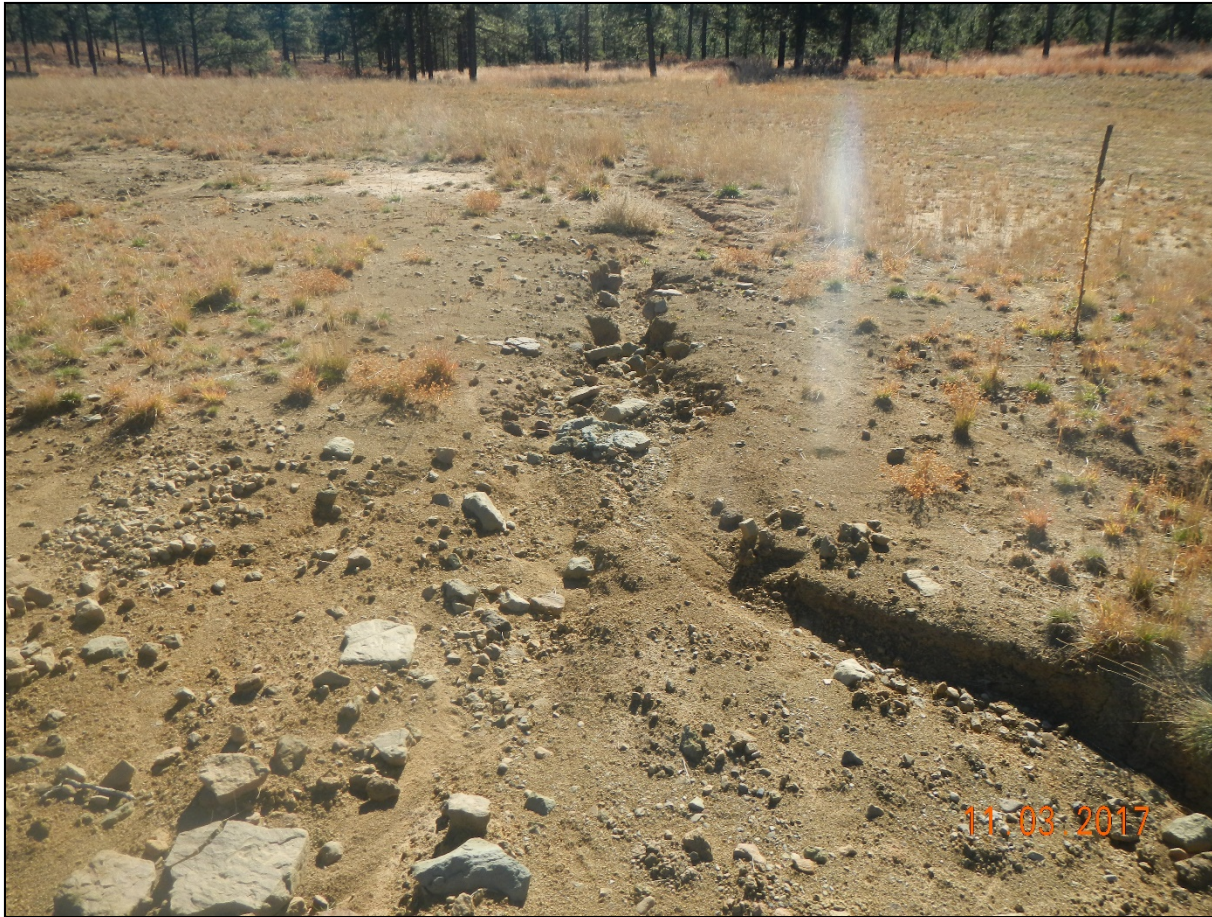
Photo 3. Facing southeast at the location. There are signs of stormwater erosion occurring thru the location.
