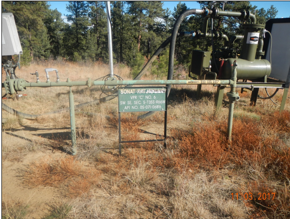
Photo 4. There is a well sign installed however the operator name and emergency contact information is faded and not legible.
