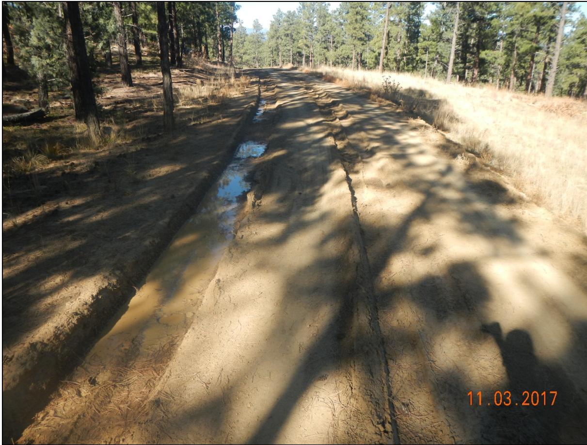
Photo 2. Facing northwest along the road. There is signs of vehicle rutting and widening of the road occurring.
