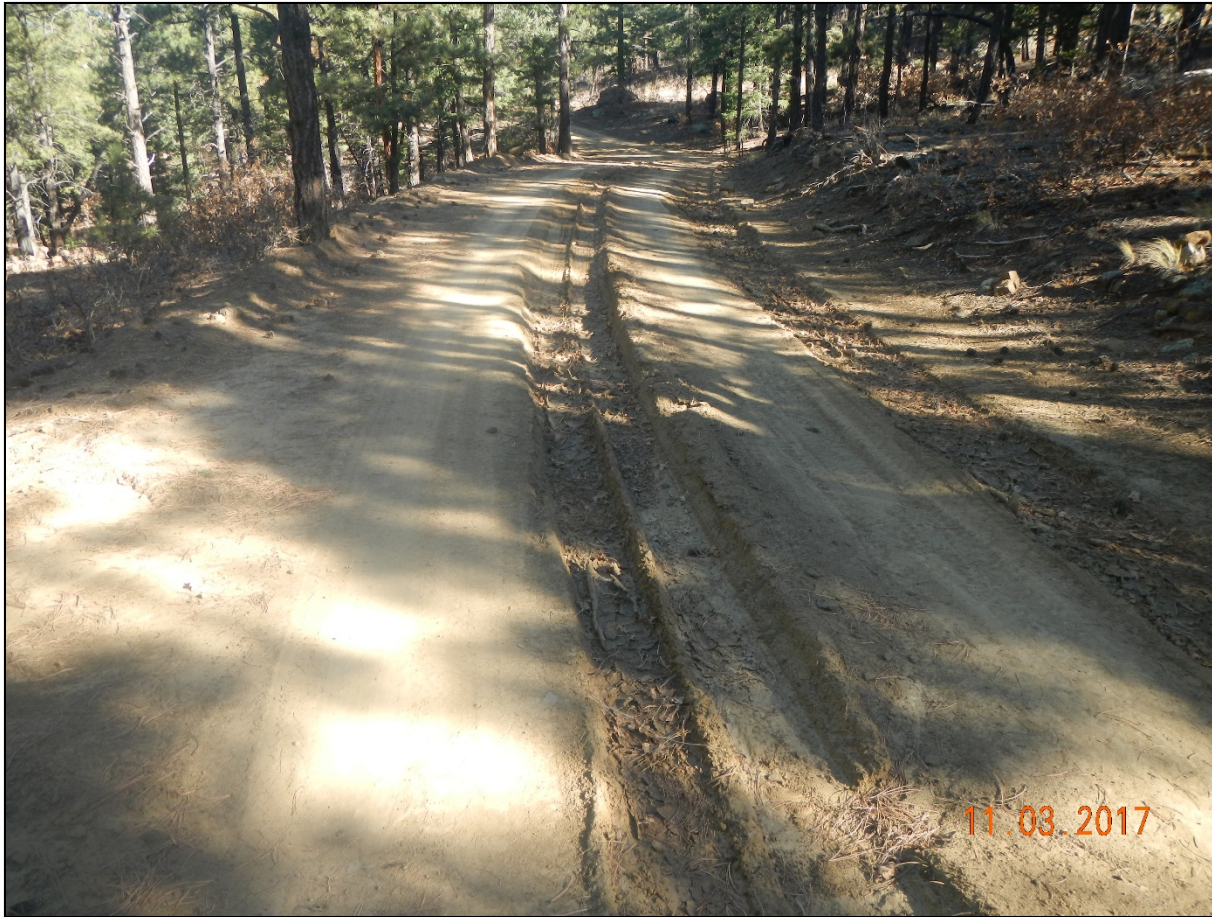
Photo 1. Facing north along the access road. There is vehicle rutting occurring along the road.
