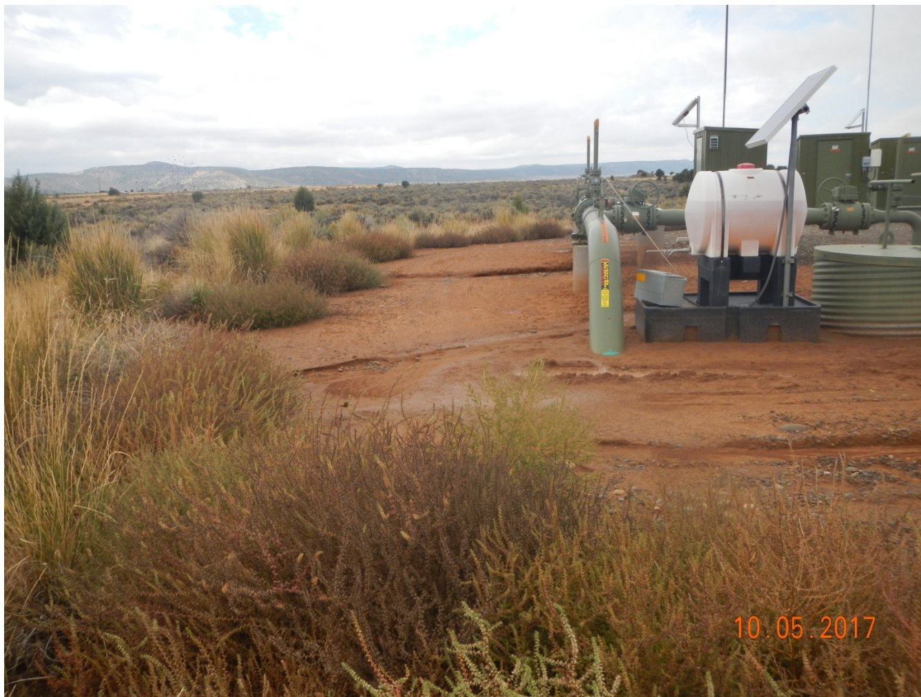
Photo 2. View of the southern portion of the project area from the well pad entrance facing westward. Erosion is occurring where runoff becomes concentrated around project facilities and flows off the well pad.
